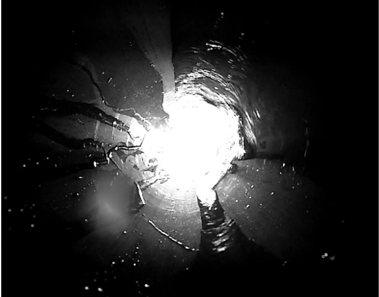
Figure 3-6 Wetting of the drain pipe at the transition region of the drain pipe observed inside a 7.6cm diameter DWHR system at a flow rate of 4 LPM.
