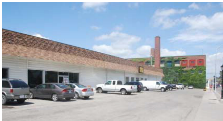
● 1.9. 50 Victoria Street North is a one-storey commercial building 9
