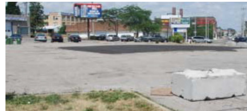
1.8. 510 King Street west which was a one-storey commercial building which was recently demolished. 8
