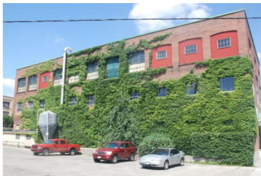
● 1.10. 60 Victoria Street North is a three-storey former industrial building (Rumpel Felt), which is currently unoccupied. It is considered a heritage building that the Region would like to see preserved and adaptively reused. 10
