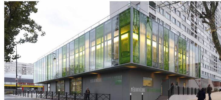
Figure 4.5 - "Arthur Rimbaud Media Library + Cultural Center". By Dacbert Cochet Chapellier Architects. 2010. Antony, France.
