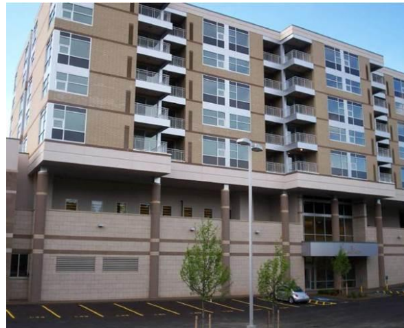
(b) five-storey CFS residential units built on an existing two-storey retail building
