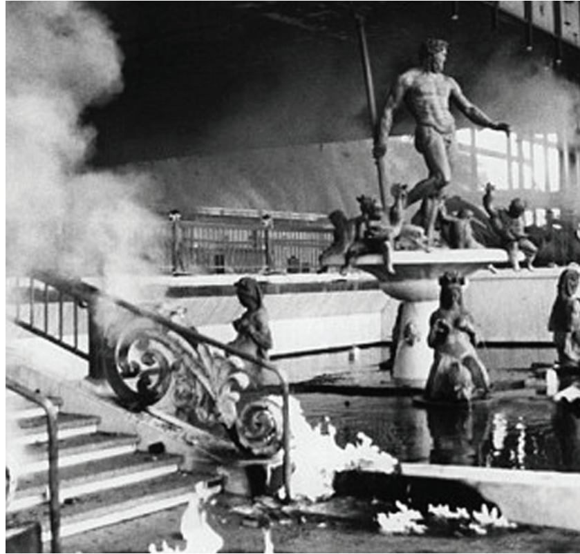
Figure 31: The original MGM Grand Hotel and Casino portecochère following an early morning fire that claimed the lives of 87 people (November 21, 1980). Associated Press
