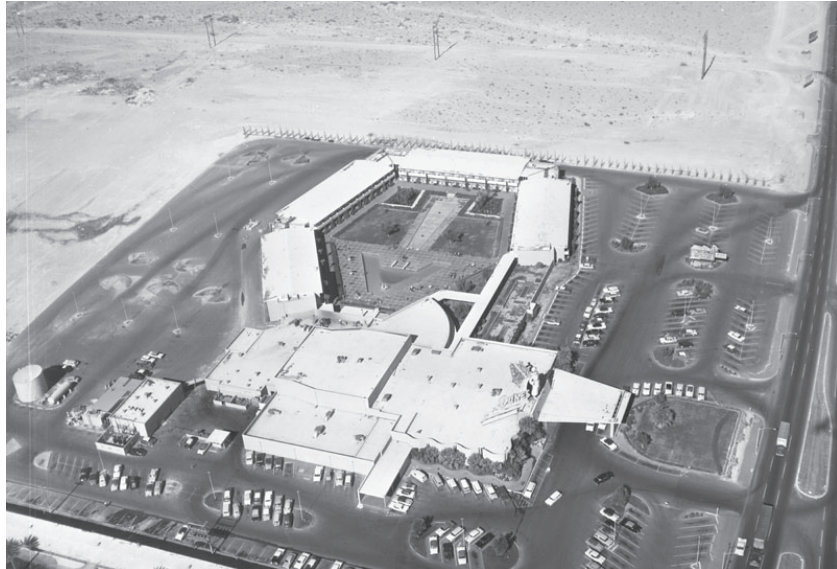
Figure 22: The Dunes motor coach building typology (1959). Kelly-Holiday Collection, Los Angeles Public Library.
