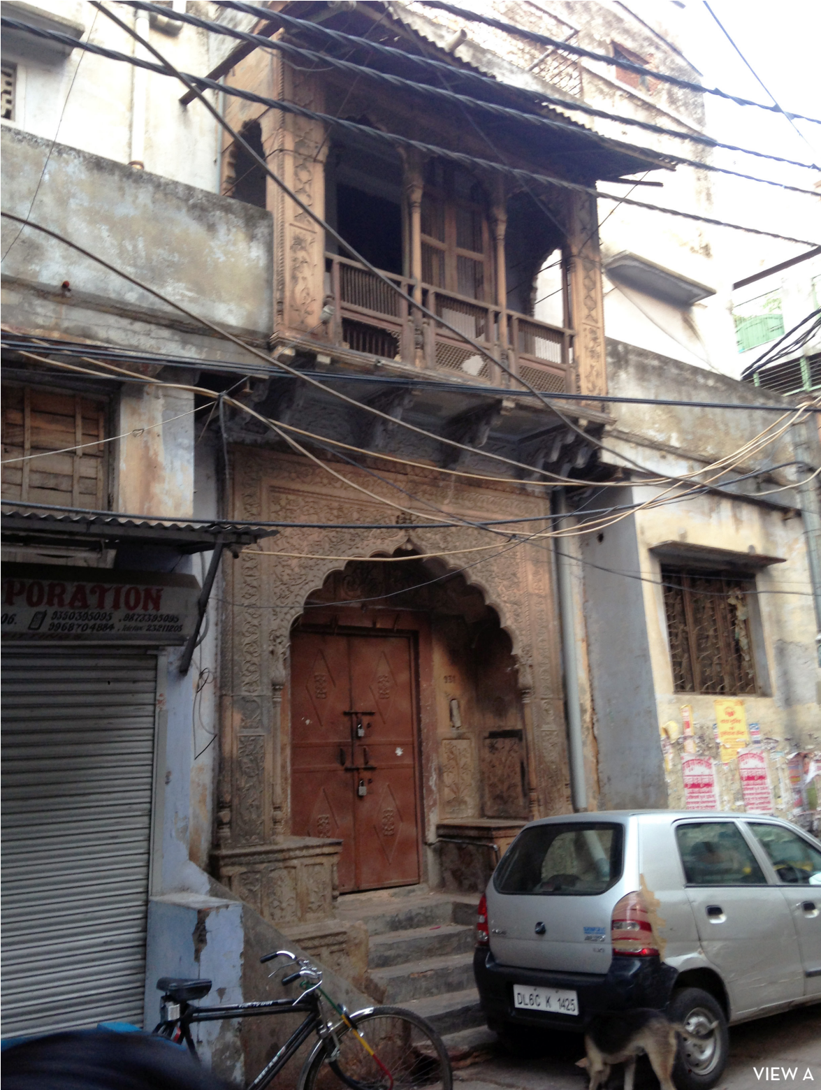
[ FIG. 4.17 ] Most of the houses have a high plinth that is approached from either sides or from the front.
