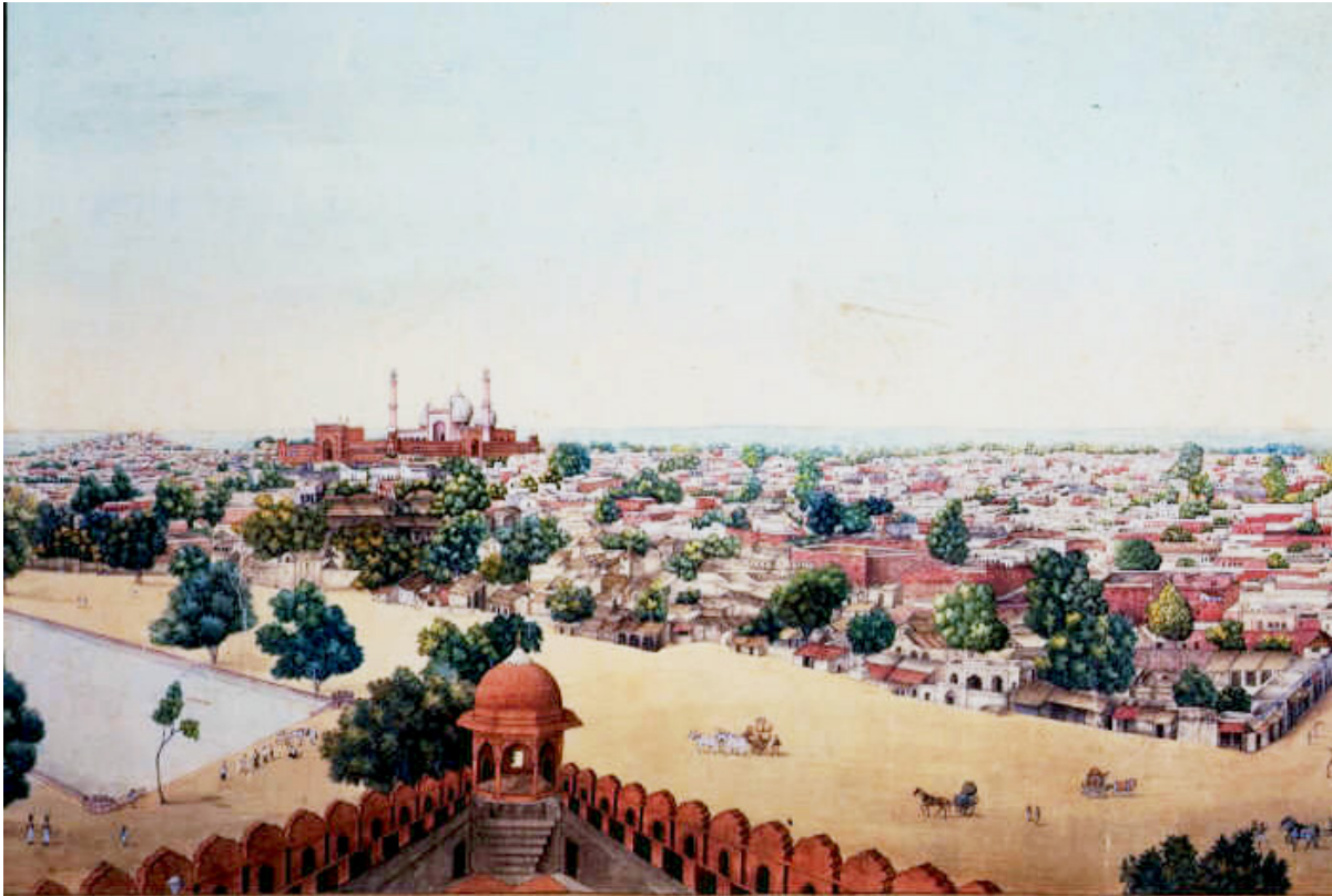
[FIGURE 2.2] View of the city from the 'Red Fort' - Looking south- west 1823 Source : British Library, New Delhi
