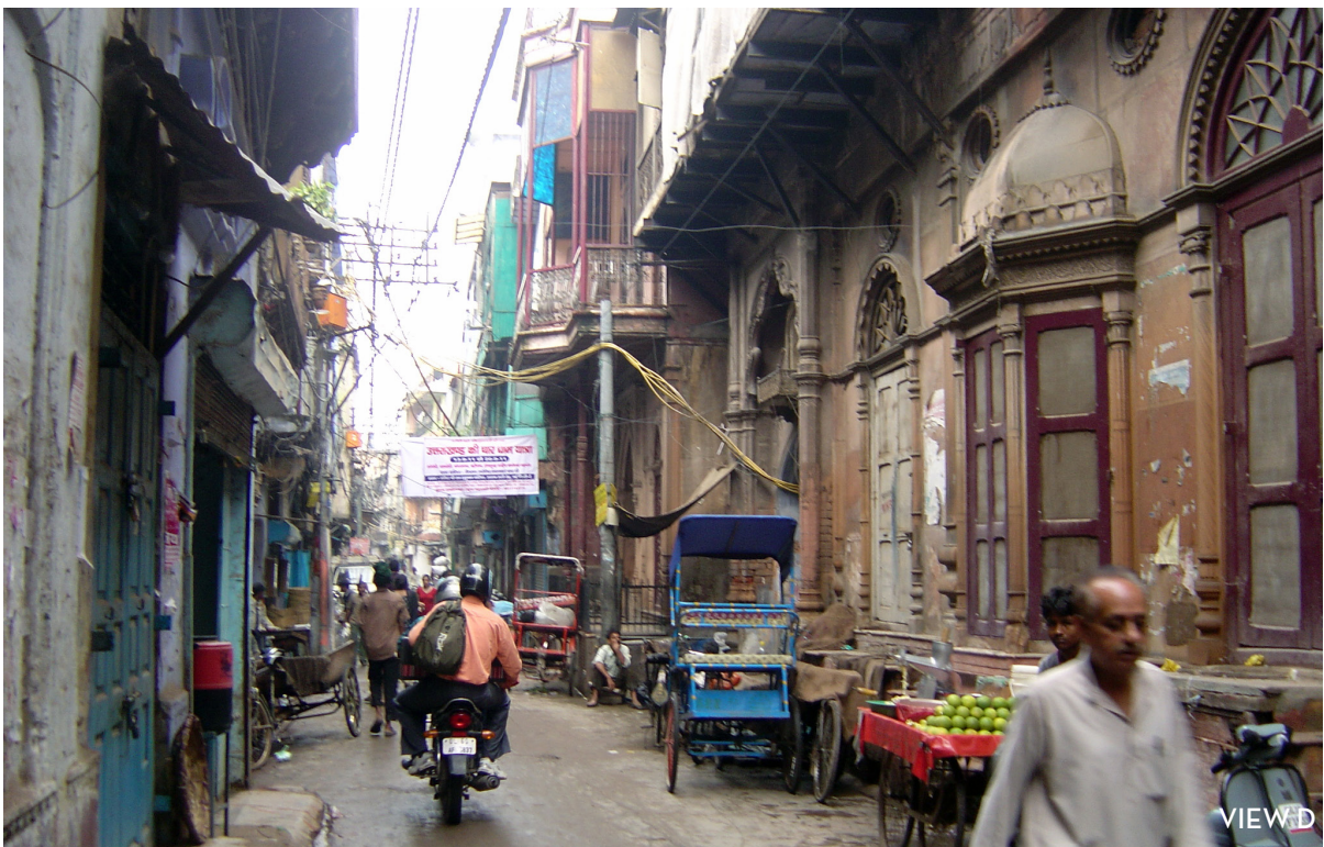
[ FIG. 4.20 ] Shops on the lower levels are now being used as godowns which is drastically changing Old Delhi
