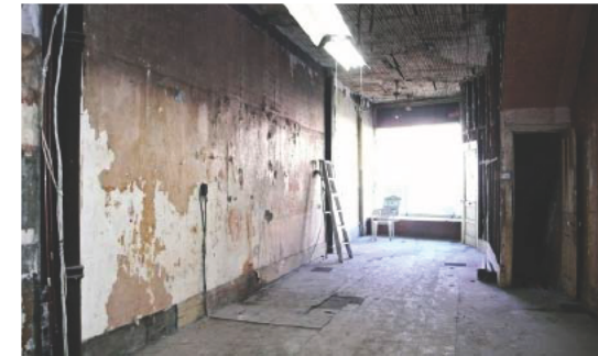
Fig. 2.2.5.5: Existing storefront and building pre-renovation (above)
