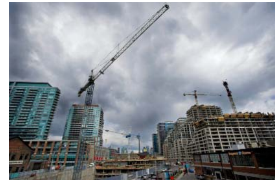
Fig. 3.1.3: State of high-rise construction in Toronto, 2014 (above)
