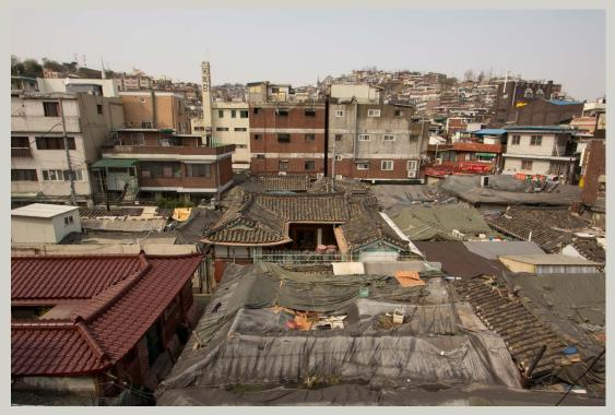
Figure 3.19 An assembly of Urban Han-Ock. There is little space between them, except for narrow alleys. Most roofs are old and in poor condition. Covered by sheets to prevent leakage during rains, the sheets indicate the extended interiors below, where outdoor courtyards used to be.
