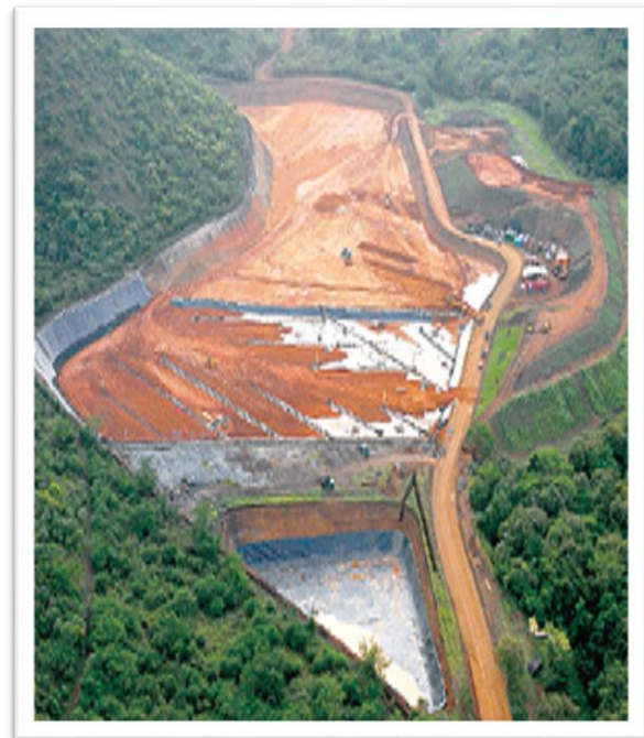
Figure D.3 Panoramic new landfill
