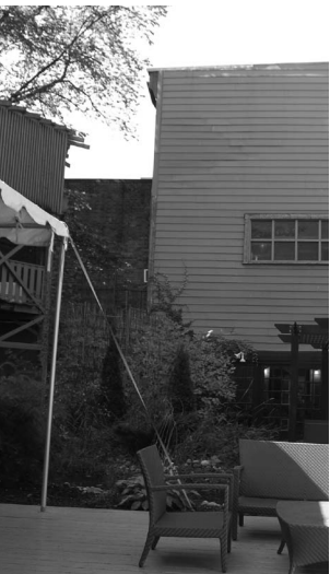
concrete and wood
