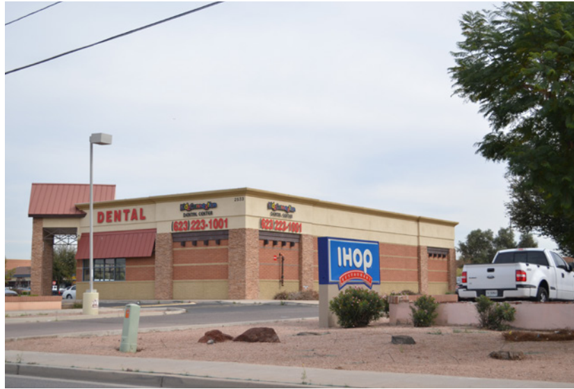
fig-60 IHOP Restaurant and Dental Office on N 75th Avenue.
