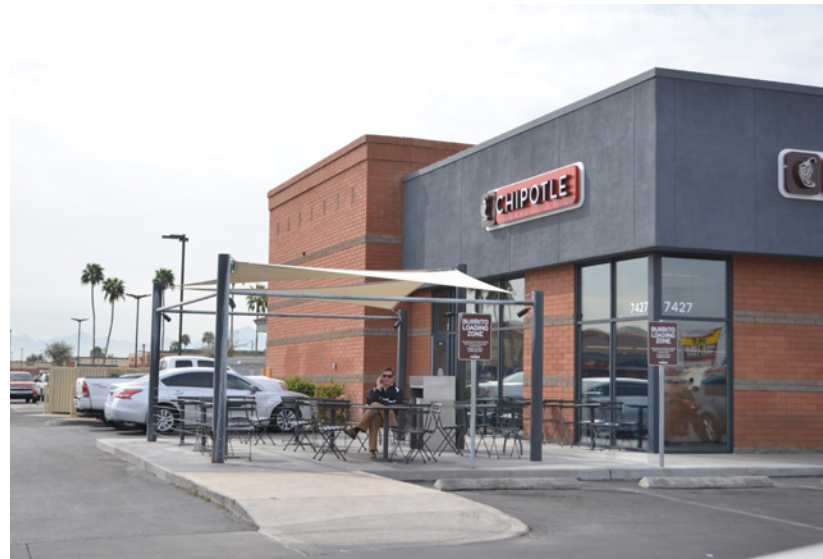
fig-53 Restaurant Patio on W Thomas Road.
