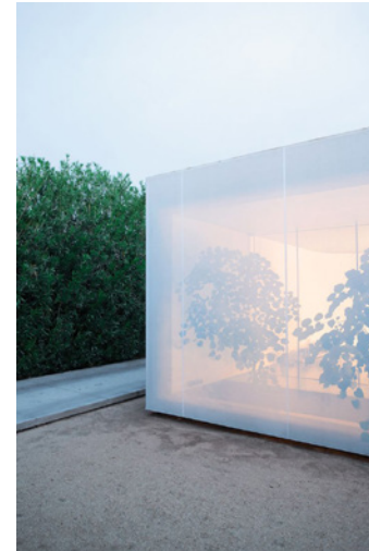
fig-106 Atherton-Keener Meadowbrook Residence Phoenix, Arizona, 2010 Ferrari shade sails stretched on steel frames become translucent when illuminated from the interior. Plants on the inside are ghosted but visible from the outside.
