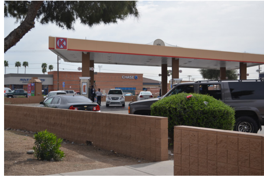
fig-56 Gas station at W Thomas Road and N 75th Avenue.
