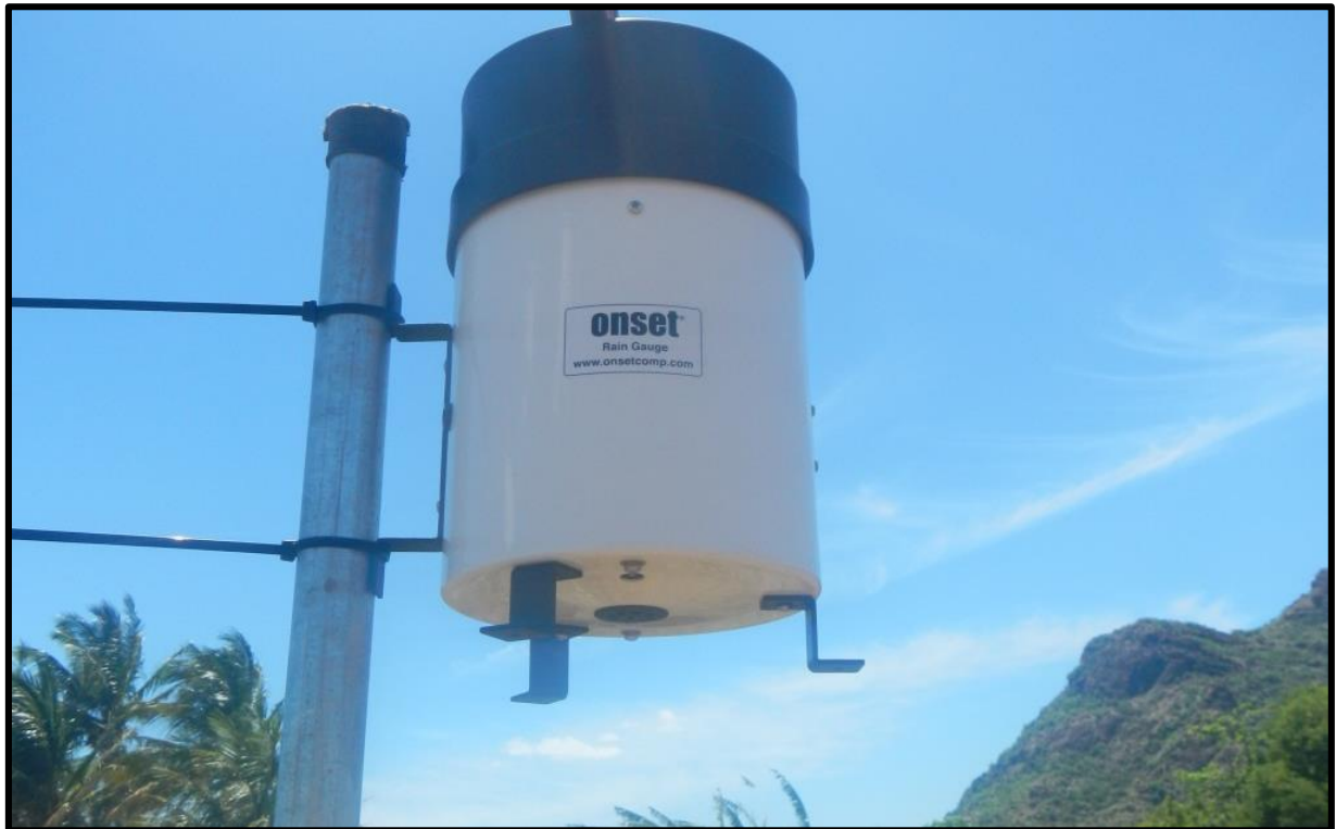
Figure 3.2: Field installation of Onset RG3-M rain gauge (Automatic tipping bucket) fixed via zip ties to 1” diameter metal pipe.
