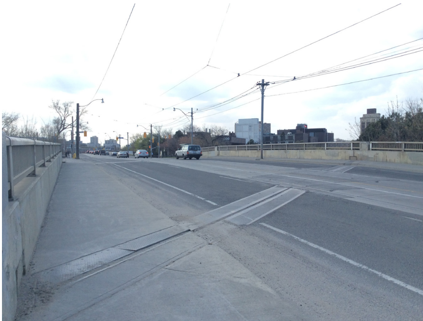
fig. 66 Dundas St W bridge / view looking northwest from Dundas St W
