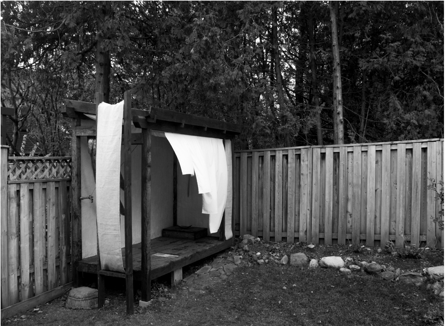
Tea Pavilion (post-renovation)
