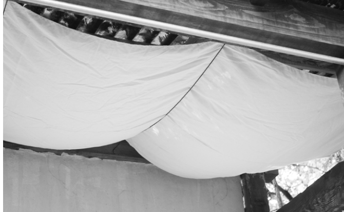
Fabric Ceiling Fig. 3.22
