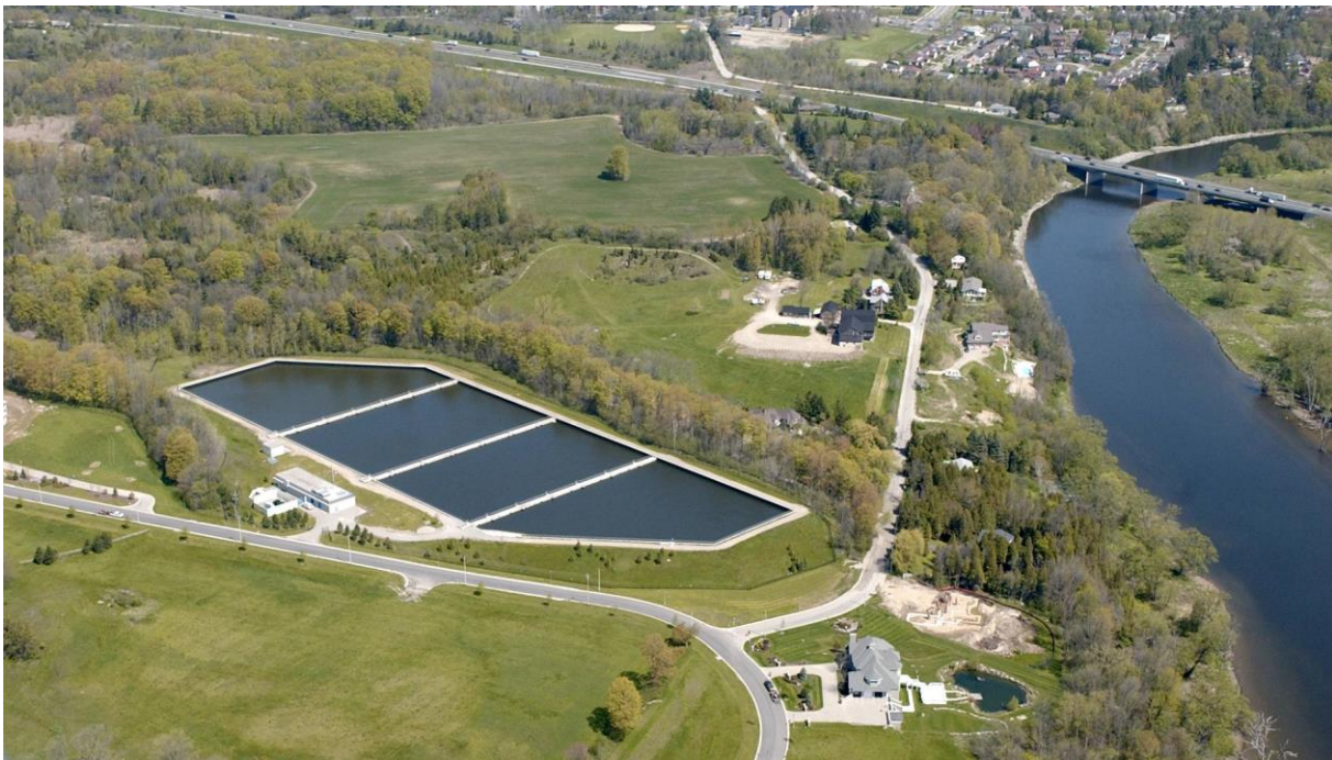
Figure 3.3: Hidden Valley High Lift Pumping Station and Grand River, Kitchener, Ontario
