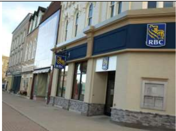
Immediately After Tornado (September 24, 2011)
