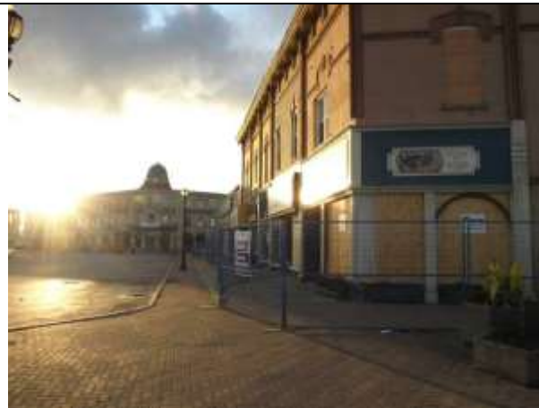
Immediately After Tornado (September 24, 2011)
