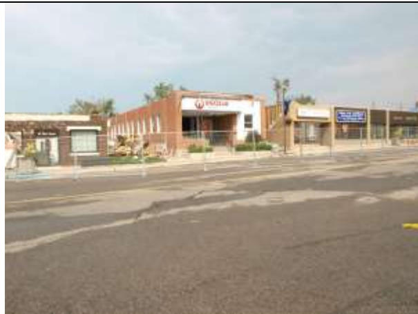
Immediately After Tornado (September 3, 2011)
