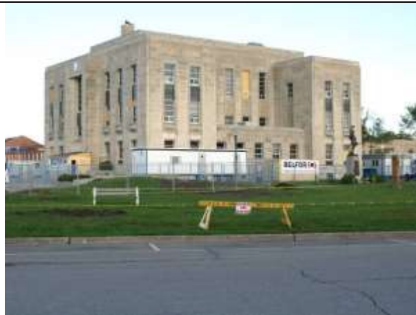
Immediately After Tornado (September 24, 2011)
