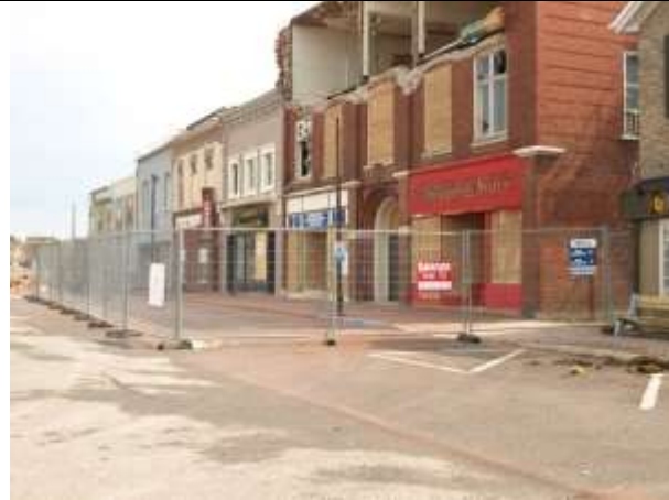
Immediately After Tornado (September 3, 2011)
