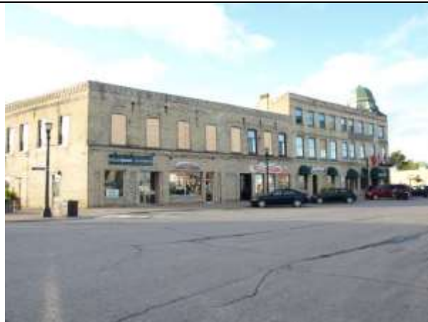
Immediately After Tornado (September 24, 2011)
