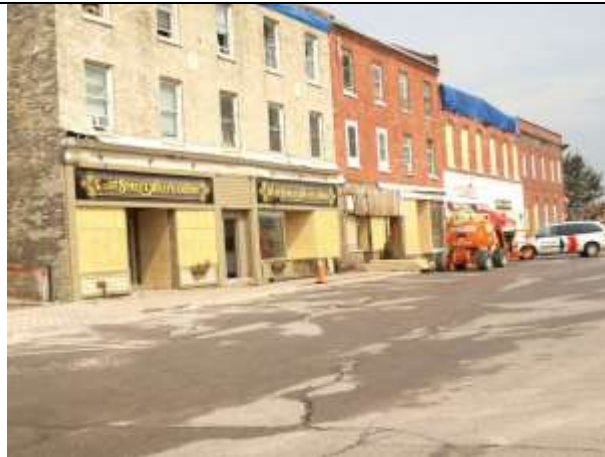
Immediately After Tornado (September 3, 2011)
