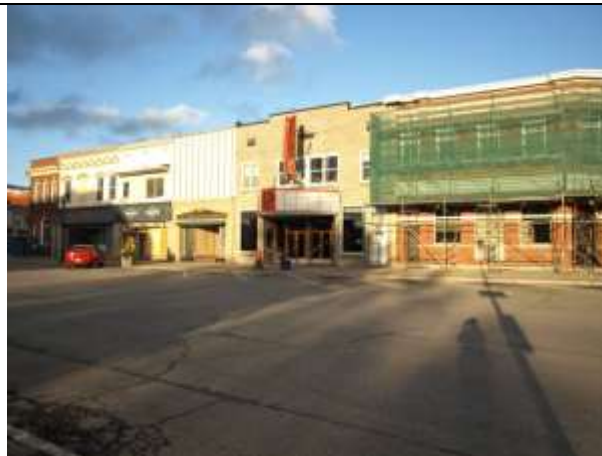
Immediately After Tornado (September 24, 2011)
