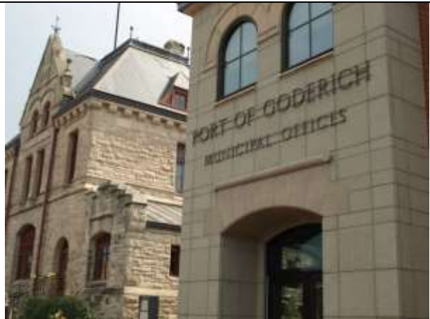
Immediately After Tornado (September 3, 2011)
