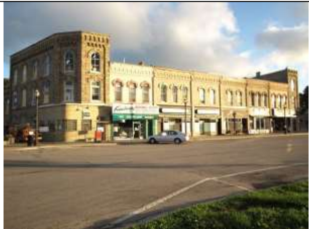
Immediately After Tornado (September 24, 2011)
