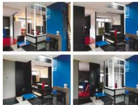
The Rietveld-Schröder House uses sliding wall partitions to divide and open up spaces. Gerrit Rietveld and Truus Schröder, 1924.
