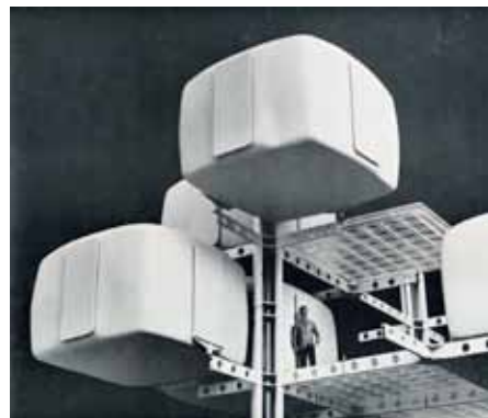
The Tekkto System offers adaptable living space as modules are joined or separated from neighbouring units. Ernest J. Kump, 1970.
