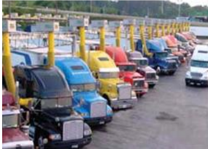
Figure 2-1: Truck stop electrification (TSE) station: an example of off-board stationary anti-idling technologies [16].
