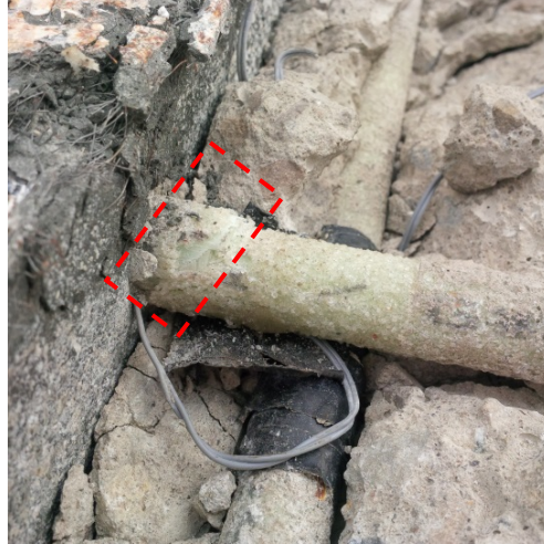
Figure 4-94. SB-3: Shear failure of top longitudinal GFRP bar after punching failure.
