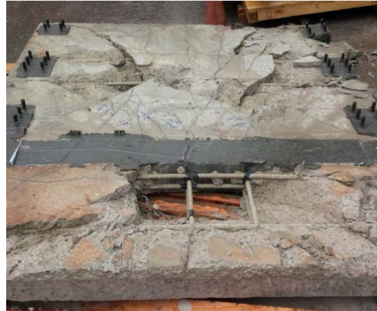
Figure A-5. SB-3: Underside of slab following concrete removal.
