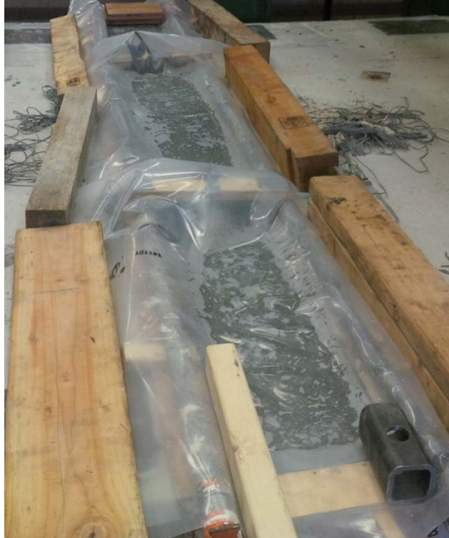
Figure 3-9. UHPC filled closure strip left covered during curing.
