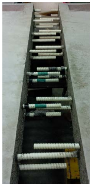
Figure 3-5. Closure strip with bars overlapped prior to UHPC casting.
