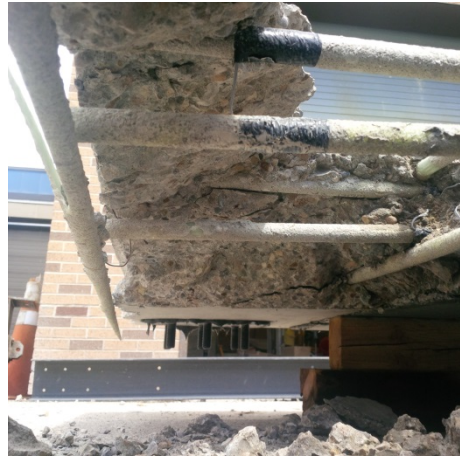
Figure A-33. SB-1: Underside of punch location with concrete removed.
