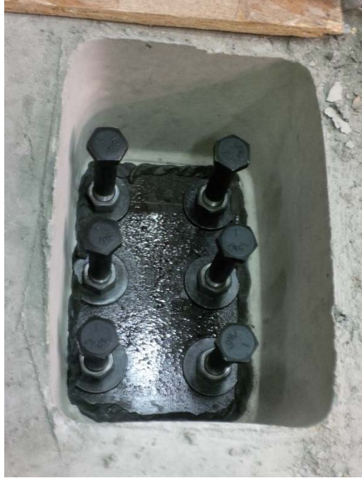
Figure 3-10. Shear bolts within pocket prior to being filled with UHPC.
