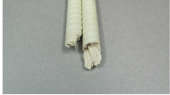
Figure A-16. RB-3: Bottom Bar #5 fracture plane.
