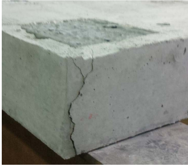
Figure 4-52. SB-1: Corner cracking occurred during failure loading adjacent to closure strip.
