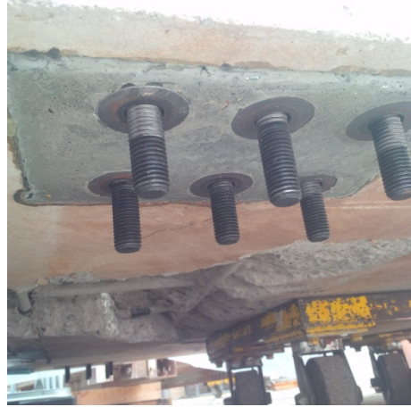
Figure A-4. SB-3: Underside of shear pocket.
