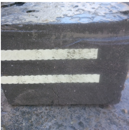
Figure A-39. RB-1: Cut through longitudinal bars in UHPC closure strip.
