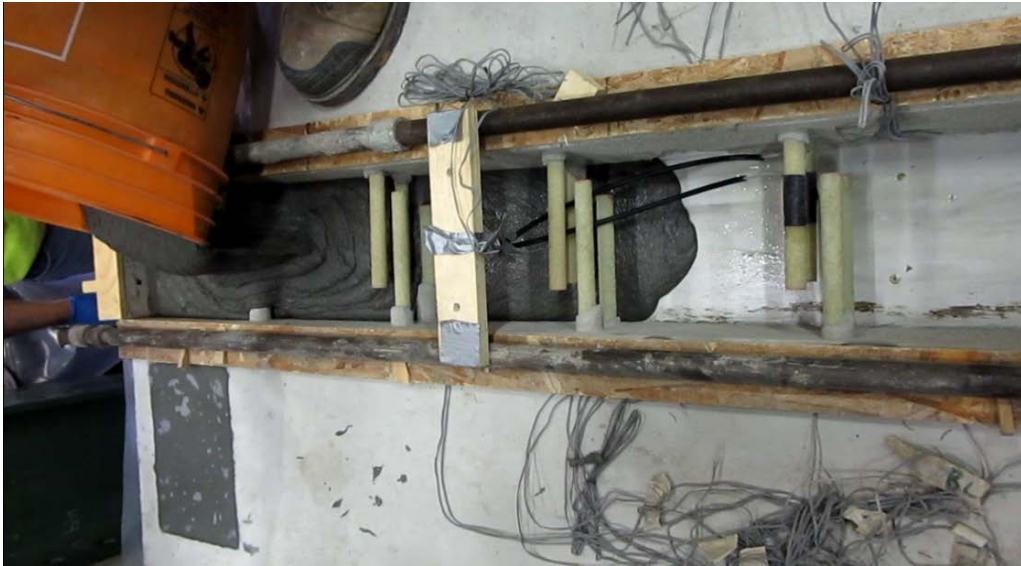
Figure 3-8. Pouring of UHPC into the closure strip.
