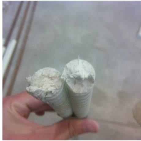
Figure A-47. RB-1: Bottom Bar #4 fracture surface.
