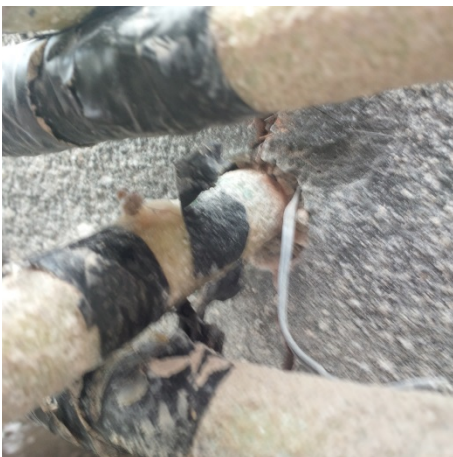
Figure A-3. SB-3: Bottom matt after punched concrete removal.
