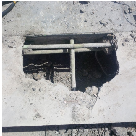
Figure A-35. SB-1: Top view of punch location with concrete removed.
