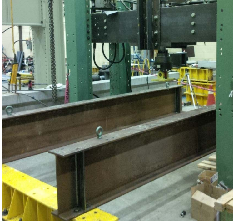
Figure 3-12. Support system prior to slab installation.
