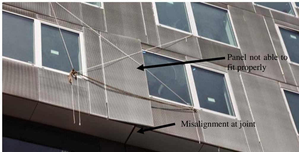
**Figure 4: Misalignment of modules at joints on B2 BKLYN building (photo used by permission of Norman Oder, Atlantic Yards/Pacific Park Report)**
