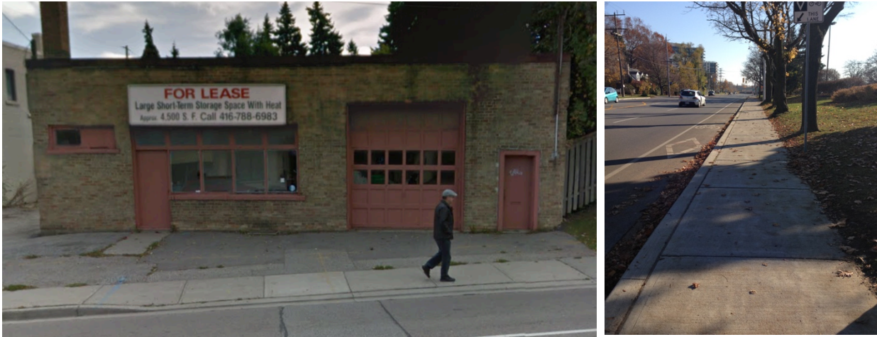
Figure 43: Abandoned Building on Segment E12, Dundas Street West (Google Maps, 2016)
