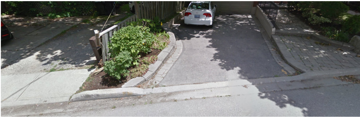
Figure 39: Discontinuous and Uneven Sidewalk on Segment E16, Walford Road (Google Maps, 2016)
