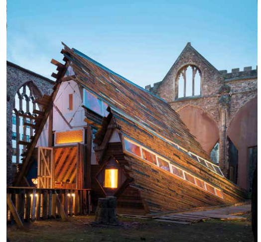
Figure 8.7: Sanctum by Theater Gates in Bristol, UK is built from reclaimed elements such as wood siding, bricks, doors, and windows.
