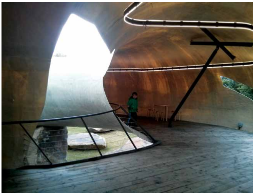
Figure 4.13: Serpentine Pavilion showing thinness of fiberglass enclosure and a continuing fascination with lightness.
