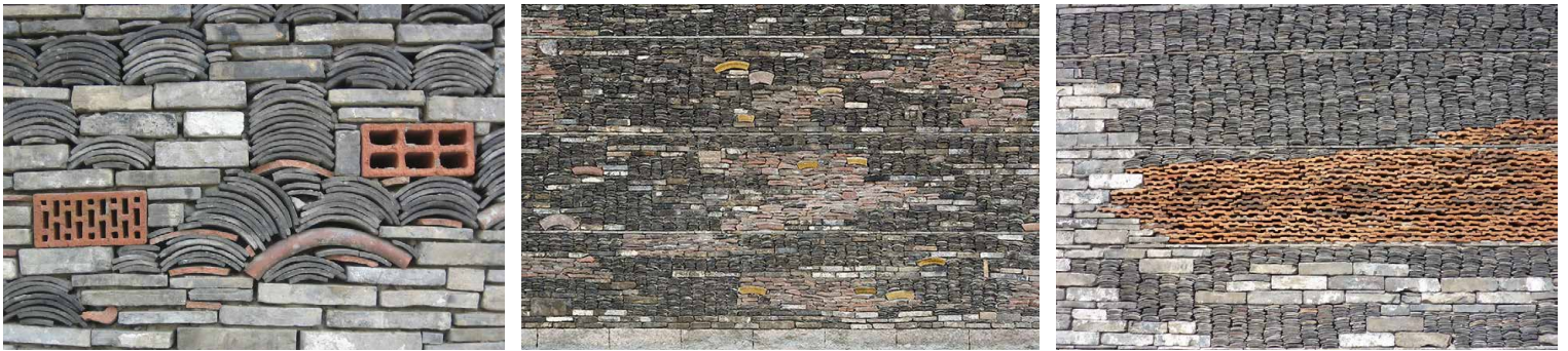
Figure 9.12: Examples of tile combinations on the Ningbo Museum facade. (1, 2, and 3).
