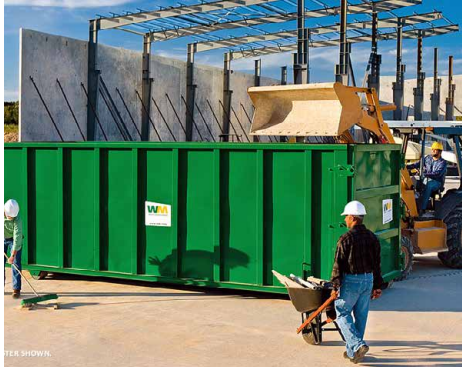
Figure 6.10: Waste collection from a construction/demolition site
