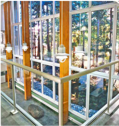
Figure 12.1: The C. K. Choi Building by Matsuzaki Architects Inc. in Vancouver, BC, was completed in 1996. 100% of the exterior brick is reclaimed, and 50% of other building materials are reclaimed or recycled products. (source: http://www.aiatopten.org/node/206 )
