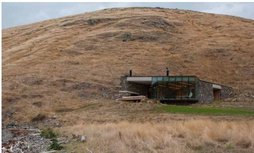
Figure 4.9: Snobetta's isolated cabin in Norway (1), a cottage on Georgian Bay by CORE architects (2), and a retreat by Patterson Associates (3) all have one thing in common: local materials and difficult to reach sites. Supplementary materials could only be brought in by horseback, boat, and four-wheel drive over a farm track, respectively.
