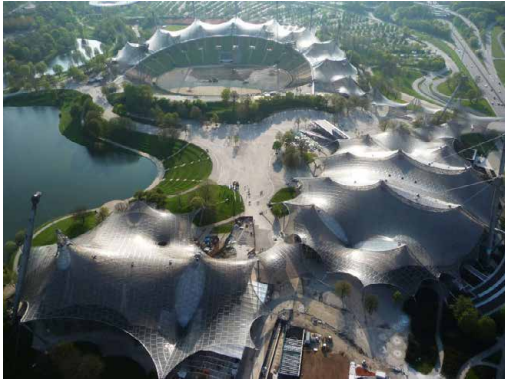
Figure 4.11: Frei Otto pioneered lightweight structures. Some of his designs were derived from studies of soap bubbles. (1) Similar to Buckminster Fuller, Otto's fascination with lightweight structures rose out of a curiosity about structural efficiency, though he recognized that just because you can build such expansive lightweight structures, they may not be needed by society and tend to be temporary. (2)
