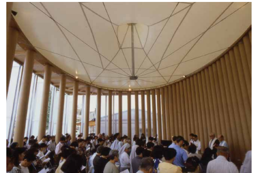
Figure 4.20: Paper Church by Shigeru Ban was a response to Kobe earthquake in 1995. After ten years of service, it was disassembled. Ban has similarly designed structures for disassembly when he knew they would be temporary, such as for exhibitions.
