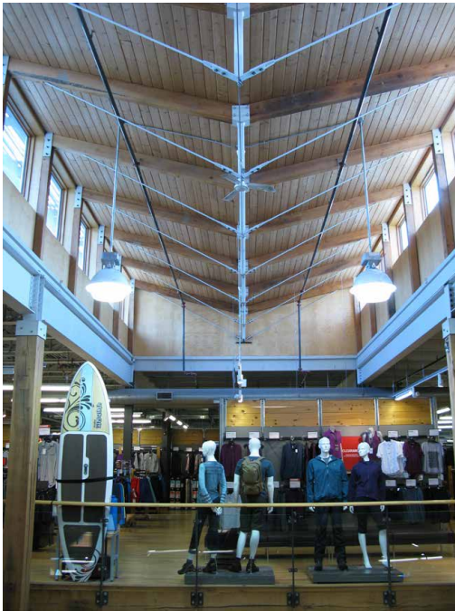
Figure 4.25: MEC Ottawa designed by architects Linda Chapman and Christopher Simmonds working with Vince Catalli and Derek Badger of by dEsign consultants. The project uses material reclaimed and reused in-situ.
