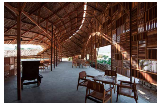
Figure 4.24: Salvaged Ring by a21 Studio in Vietnam is built with many scraps of wood from a local carpenter.
