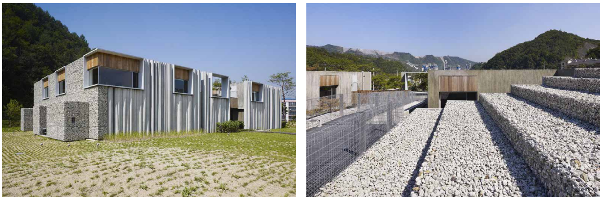
Figure 5.15: Hanil Visitors Center & Guest House by BCHO Architects uses gabion baskets filled with crushed (therefore "downcycled") concrete.
