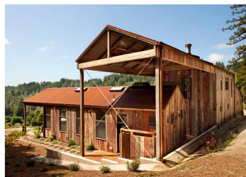
Figure 8.5: The Aptos retreat by CCS Architecture in San Francisco uses reclaimed barn wood as cladding.
