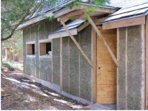
Figure 4.7: This strawbale construction office by Ingrid Cryns of Soma Earth is uses waste straw from the agriculture industry; it is renewable and local to Southern Ontario. Walls tend to be very thick.
