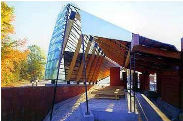
Figure 5.7: Glass Chapel/Mason's Bend Community Center by Rural Studio in Hale, Alabama reuses windshields to create a semi-enclosed space.
