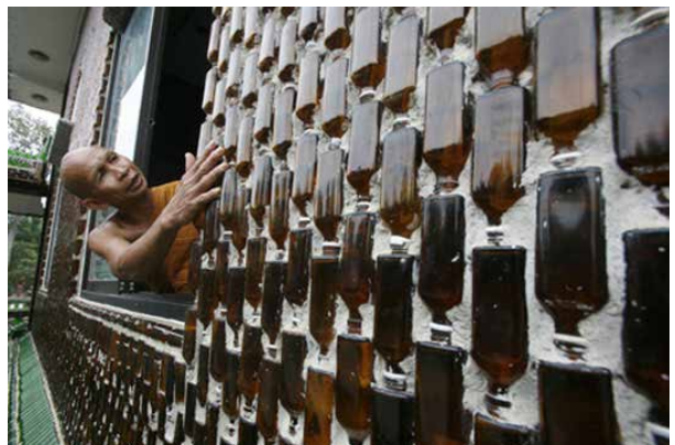
Figure 5.8: Wat Pa Maha Chedio Kaew temple in Sisaket, Thailand reuses consumer glass bottles as bricks.
