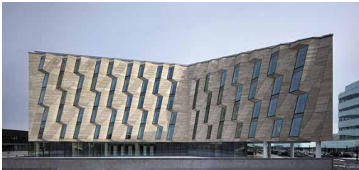
Figure 4.5: Horten Headquarters facade uses a composite of travertine and fiberglass.
