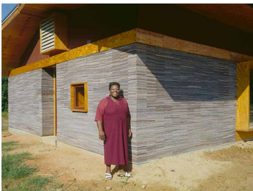
Figure 4.19: Lucy Carpet House by Rural Studio uses stacked worn carpet tiles for the walls.
