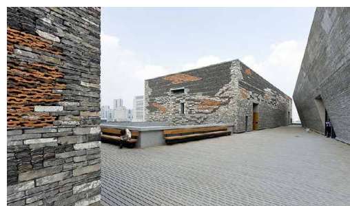
Figure 12.2: Ningbo Historic Museum by Wang Shu, Amateur Architecture Studio in Ningbo, China follows in the tradition of wapan construction by using a mix of reclaimed bricks and tiles from the demolition of historic neighbourhoods.
