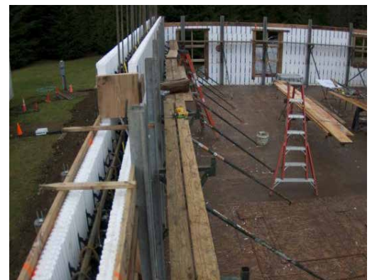
Figure 4.2: Insulated concrete forms (ICF) are a composite of insulation and spacers that act as formwork for concrete. They can speed up construction time because the insulation does double duty.
