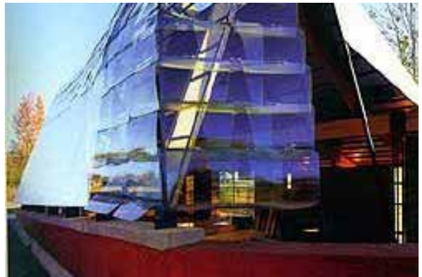
Figure 5.7: Glass Chapel/Mason's Bend Community Center by Rural Studio in Hale, Alabama reuses windshields to create a semi-enclosed space.
