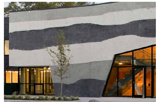
Figure 9.3: Striated concrete test on elevator shaft, wall after two pours, (1) and the finished wall. (2)
