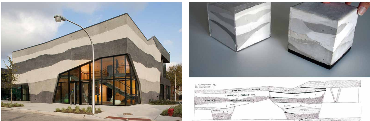
Figure 5.14: SOS Children's Village Community Center by Studio Gang in Chicago, 2008; the team used leftover readymix concrete from condominium construction sites at the end of each day to build up the exterior walls; the concrete was donated.
