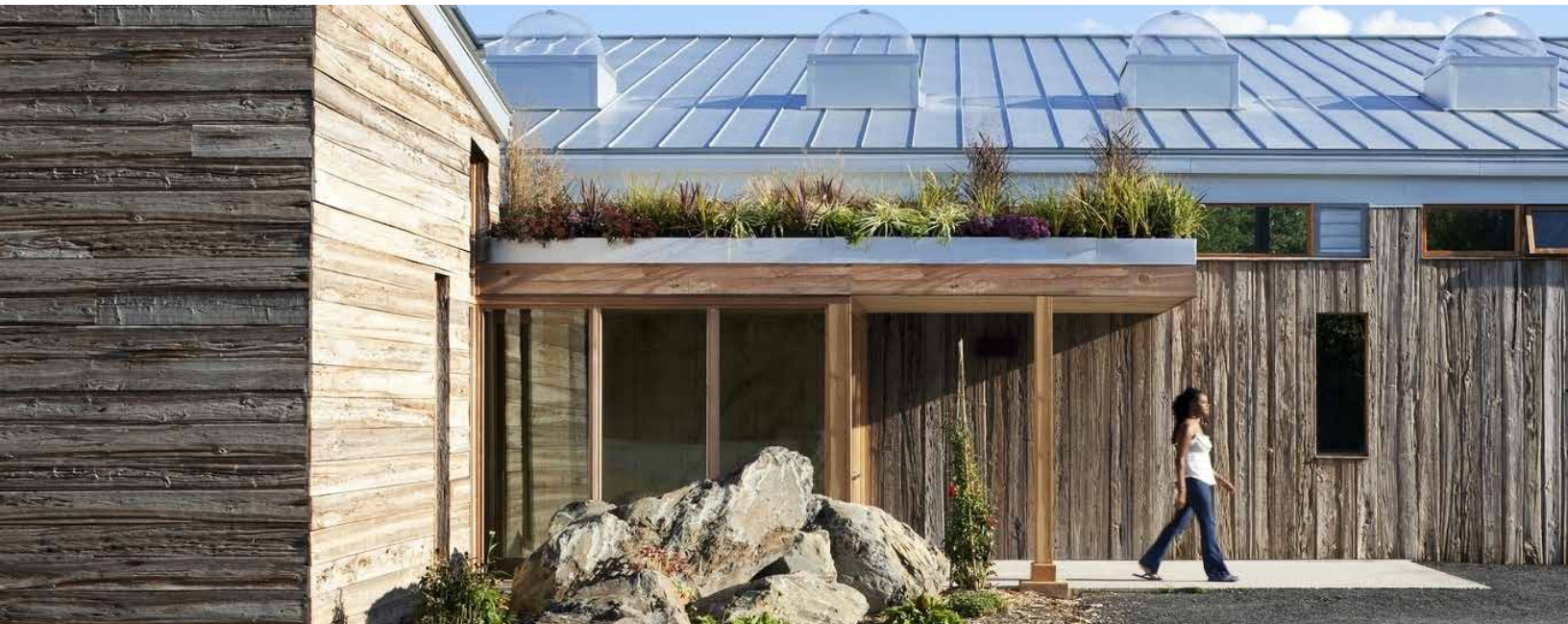
Figure 8.2: Omega Center for Sustainable Living by BNIM Architects in Rhinebeck, NY “uses cypress salvaged from mushroom farms, beech reclaimed from former factories, and planks from the 2009 inauguration platform of President Barack Obama.” (source: http://www.architectmagazine.com/technology/recycling-building-materials_o?o=1 )
