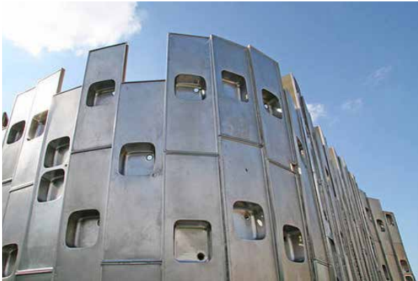
Figure 5.3: “Reycloop” kitchen sink building by Superuse Studio in Amsterdam is an installation that reuses old steel sinks.
