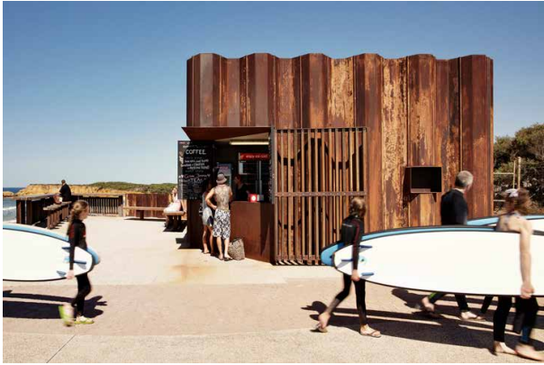
Figure 5.2: Third Wave Kiosk by Tony Hobba Architects in Australia reuses steel piles.
