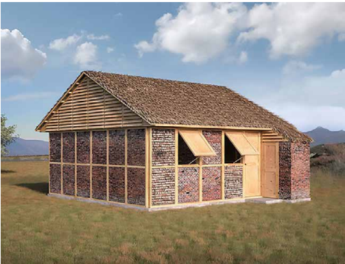
Figure 4.23: Concept design by Shigeru Ban to build relief shelters in Nepal from building rubble.
