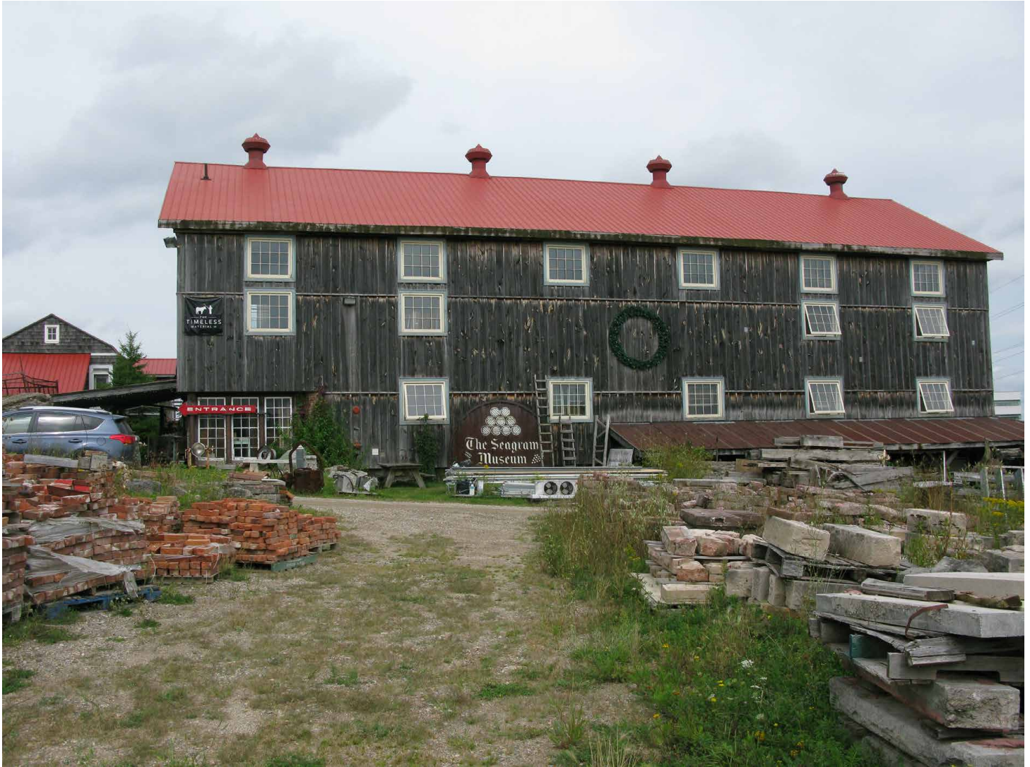
Figure 10.3: The Timeless Material Company main building
