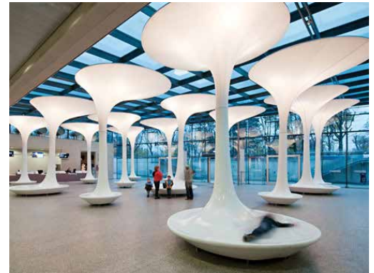
Figure 4.3: Fibre-reinforced plastic in the seating at the TMW technical museum, by Querkraft Architects.
