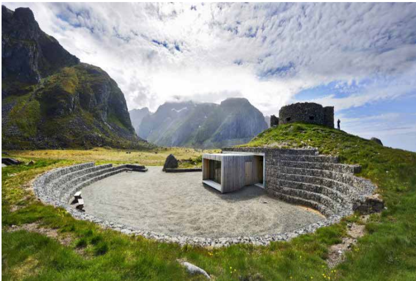
Figure 4.10: The Eggum Tourist Stop by Snobetta uses rock excavated from the site and locally-gathered driftwood.
