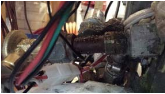
Figure 5.31 TXV without frost
