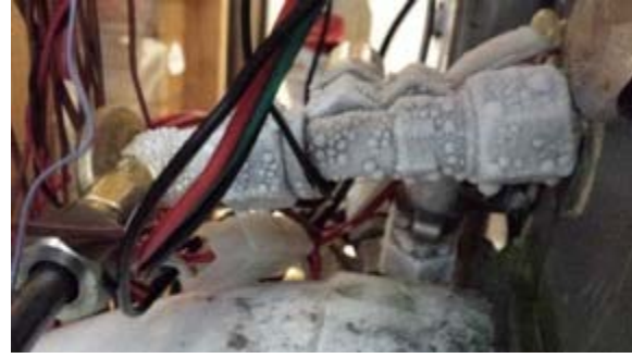
Figure 5.32 TXV with frost
