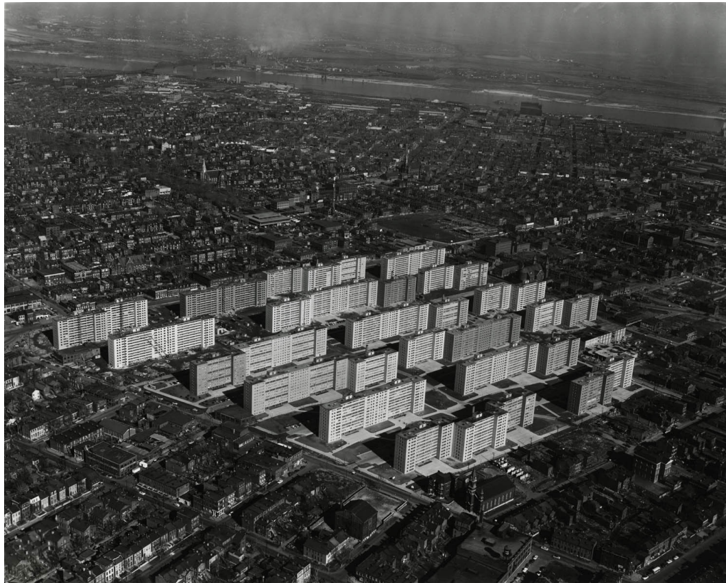
Figure 2.16- An aerial view of the Pruitt-Igoe housing project in St. Louis, Missouri shows just how alien the project seemed in comparison to its low-rise surroundings.
