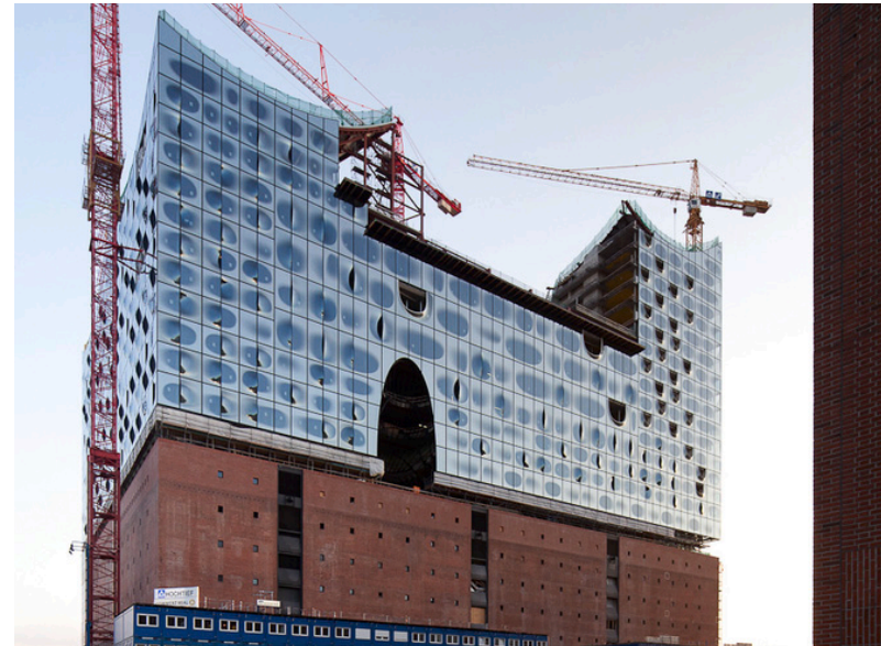
Figure 4.6- Construction photo of the Elbe Philharmonic Hall (2011).
