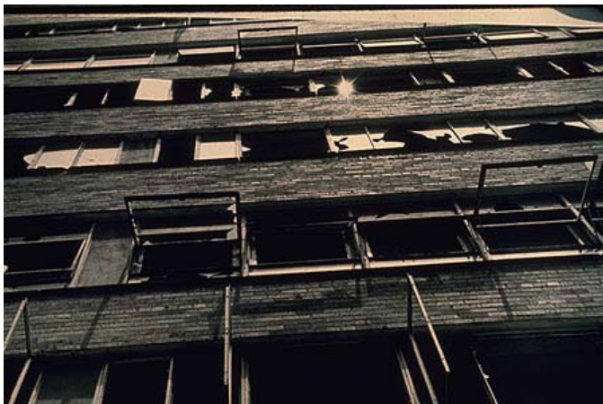
Figure 2.18- (Top Left) Interior corridor of one of the Pruitt-Igoe buildings. (Top Right) Broken incinerator inside one of the buildings. (Bottom Left) Broken windows were a permanent problem at Pruitt-Igoe. (Bottom Right) Over 10,000 broken windows resulted in frozen pipes that melted and burst, destroying hundreds of apartments. These photos demonstrate the lack of maintenance that resulted in the rapid deterioration of the Pruitt-Igoe housing project.
