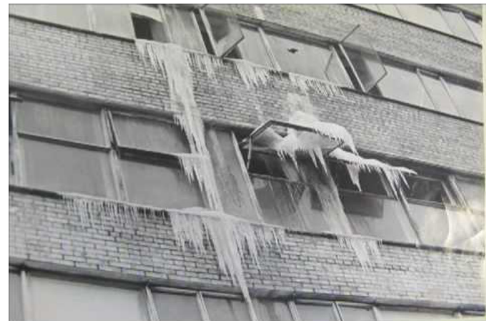
Figure 2.18- (Top Left) Interior corridor of one of the Pruitt-Igoe buildings. (Top Right) Broken incinerator inside one of the buildings. (Bottom Left) Broken windows were a permanent problem at Pruitt-Igoe. (Bottom Right) Over 10,000 broken windows resulted in frozen pipes that melted and burst, destroying hundreds of apartments. These photos demonstrate the lack of maintenance that resulted in the rapid deterioration of the Pruitt-Igoe housing project.
