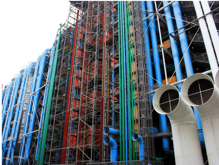
Figure 3.18- Exterior photo of the Centre Pompidou high-lighting the colour-coordinated building systems.
