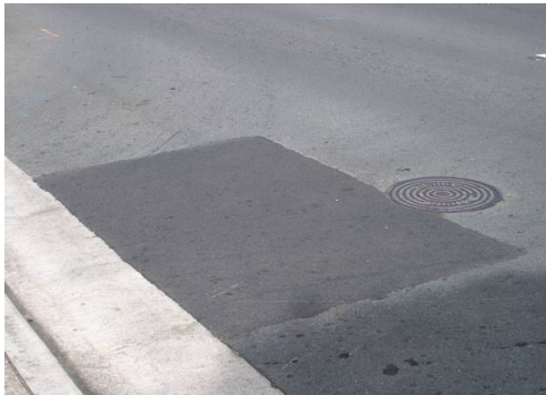
(e) Road patching [35]
