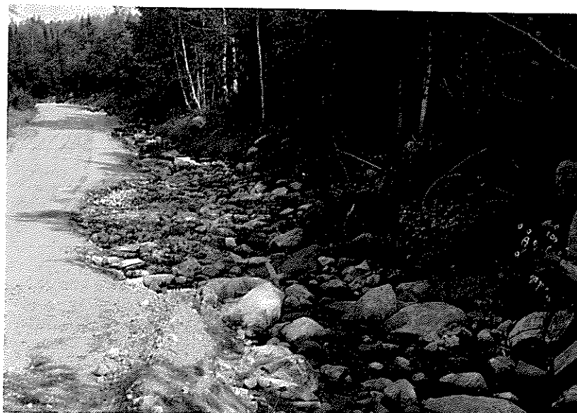
Figure 7-3 Channeling of runoff into ruts on a lumber road north of Baie Trinité. In 1972 the road occupied the right half of the road shown in the photo, and the area which is now part of the creek bed. Photo taken in 1974.
