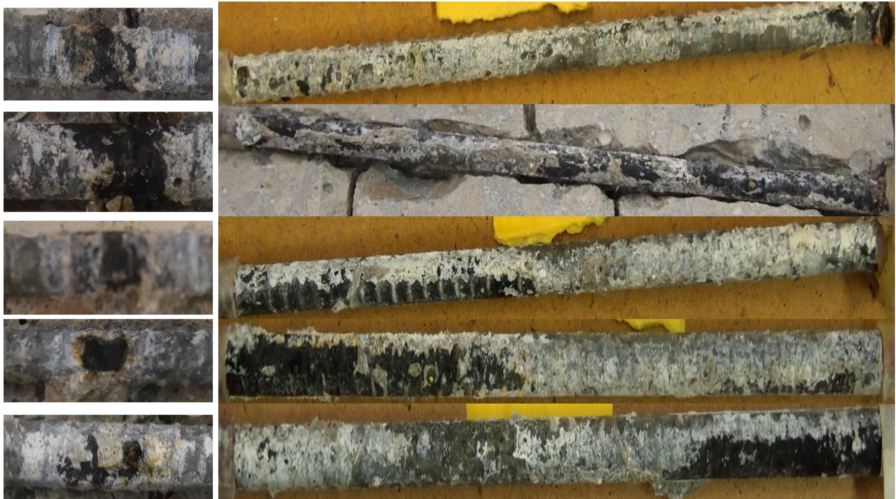
Figure E2.4.1: Exposed surface (to concrete crack) of transversely- (left) and longitudinally- (right) cracked HDG steel specimen 1 to 5.
