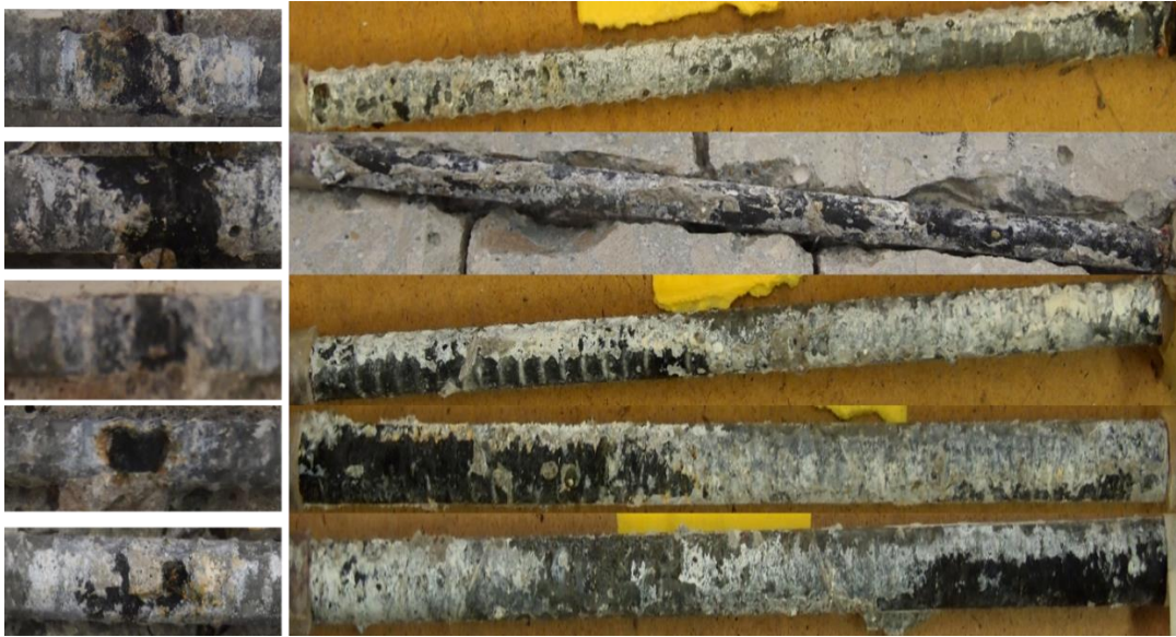
Figure 4-17: Exposed surface (to concrete crack) of bars in transversely- (left) and longitudinally- (right) cracked HDG steel specimen 1 to 5.
