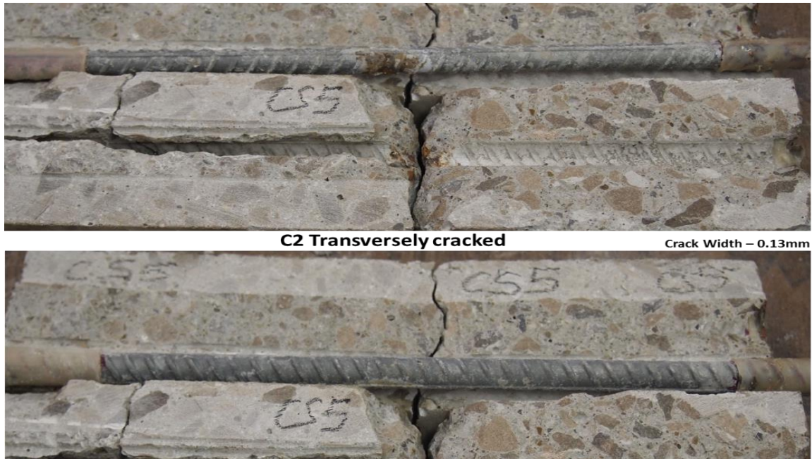
Figure 4-16: Concrete specimen of autopsied transversely cracked C2 specimen.
