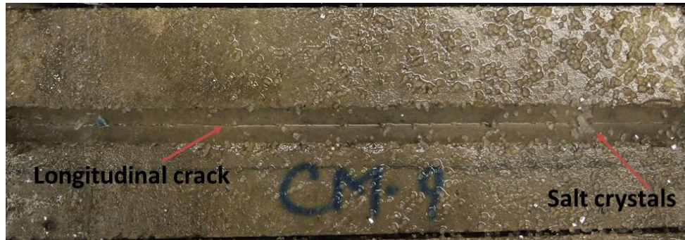
Figure 4-15: Salt crystals on the surface and in the cracked region. Such crystals in the crack could block further ingress of salt.
