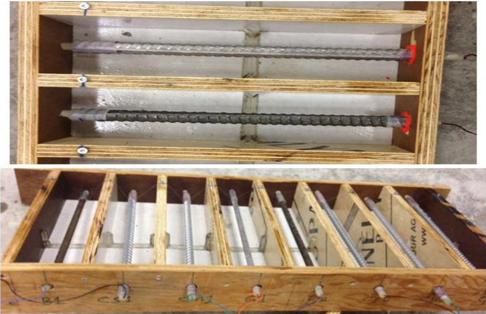
Figure 3-5: Formwork for transversely cracked specimens with rebar in place.
