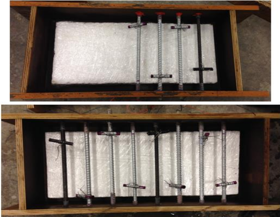
Figure 3-4: Sound beam formwork. Note: cross bars were straightened before placing concrete.
