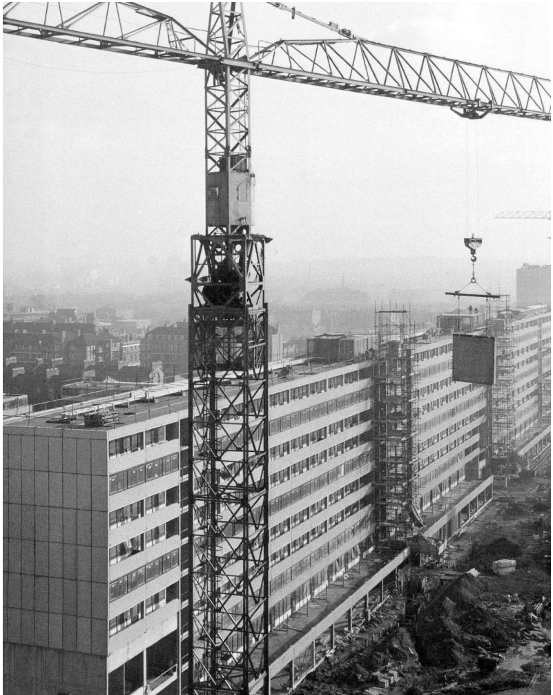
Fig 22 Aylesbury Estate under construction.
