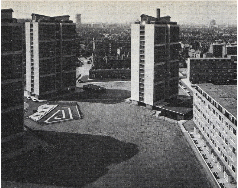
Fig 09 Brandon Estate, Ted Hollamby & LCC Architects' Department 1960.
