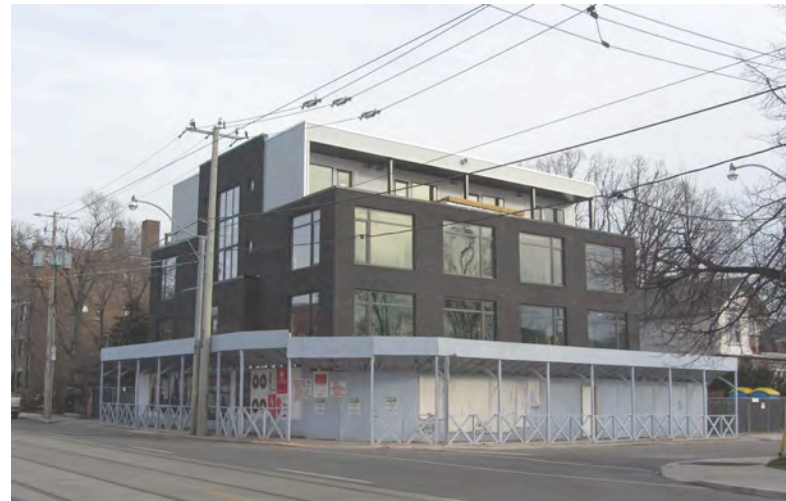
fig 3.105 Street view of the back-to-back townhouse units under construction.
