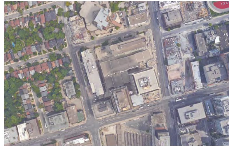
fig 3.52 Aerial photo of the project's block. Note the lot coverage and potential impact (e.g. urban heat island effect, wind, and shadow).
