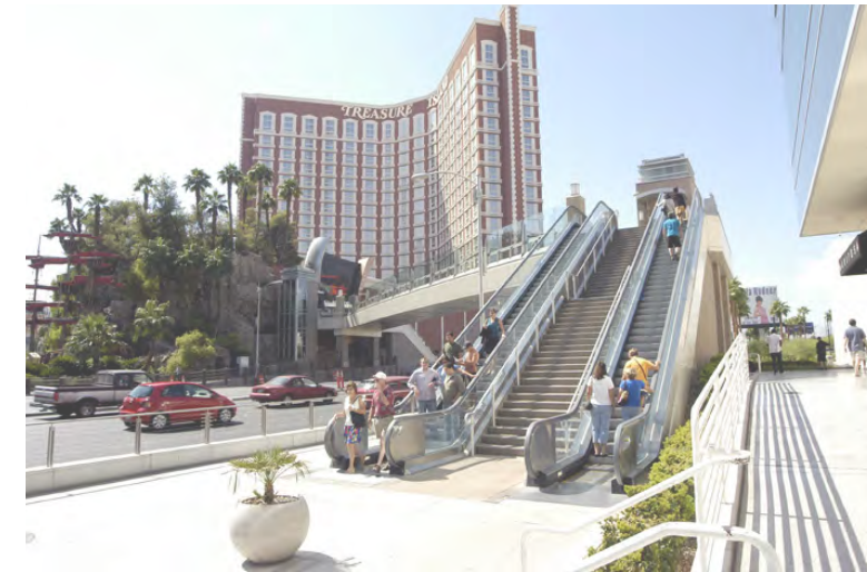
fig 5.43 Freestanding pedestrian bridge street crossing in Las Vegas.
