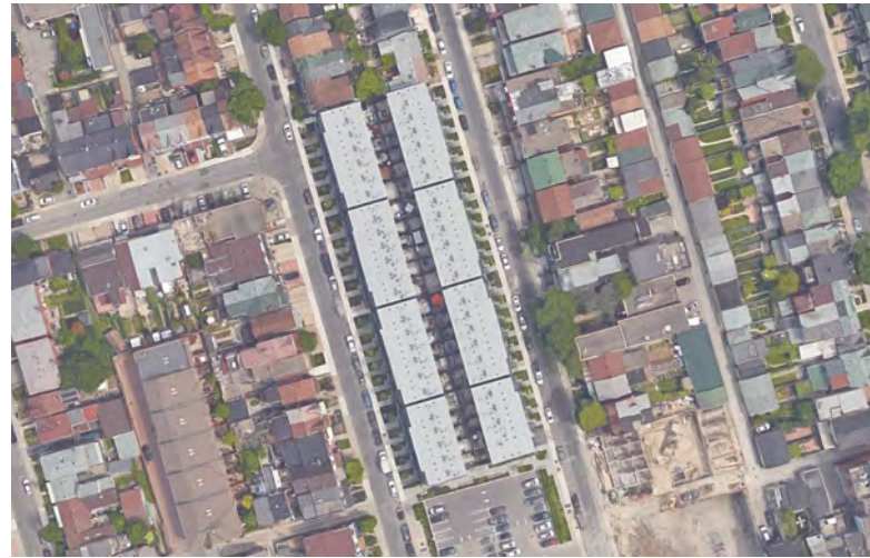
fig 3.112 Aerial photo of the project showing its infill of a traditional Toronto block width with a higher density of building.
