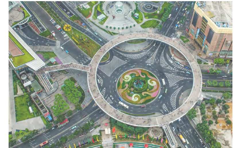
fig 5.44 Freestanding pedestrian circular bridge in Shanghai.
