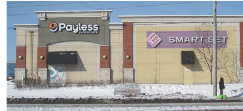
fig 2.27 Photograph of the edge-condition Eglinton near Hakim Avenue (north side).
