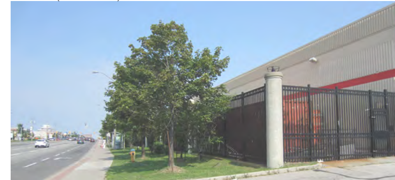
fig 2.28 Photograph of the edge-condition Eglinton near Hakim Avenue (south side).
