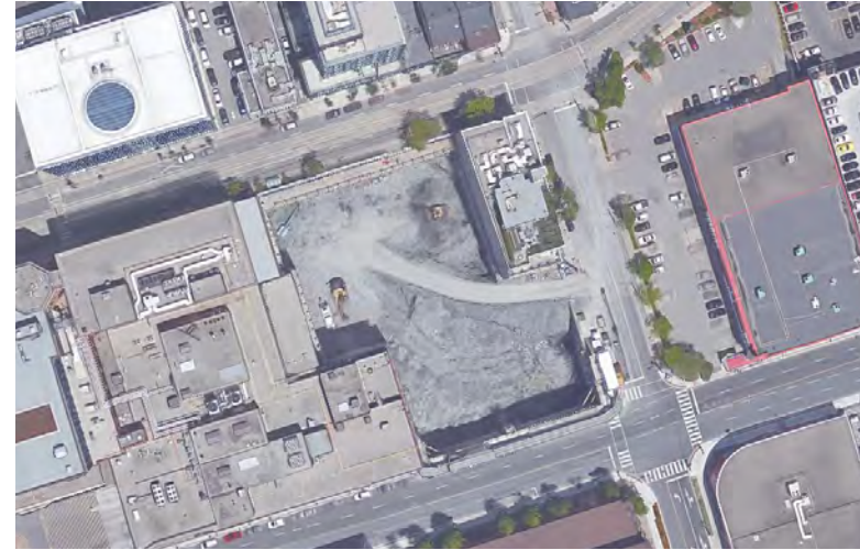
fig 3.76 Aerial photo of the project's excavated site and surrounding context.
