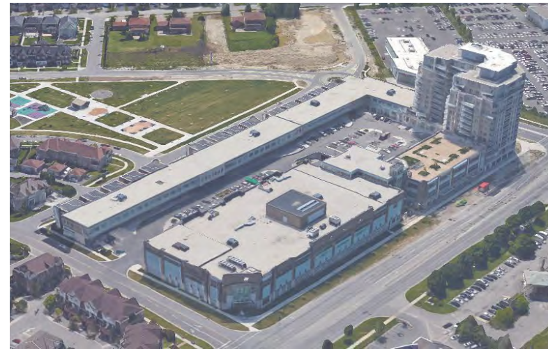
fig 3.59 Axonometric photo looking south showing the corner grocery store, mid-rise tower, and surface parking in the centre of the block.
