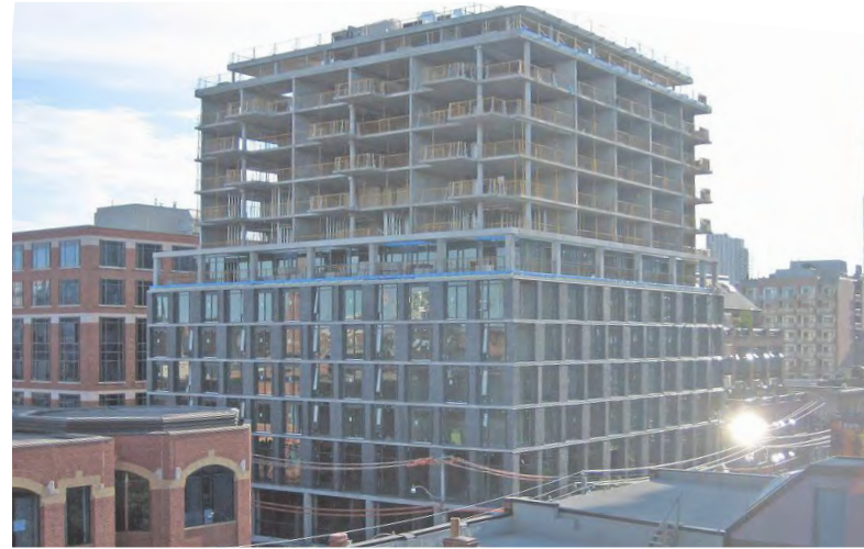
fig 3.81 Photo of the project during construction.
