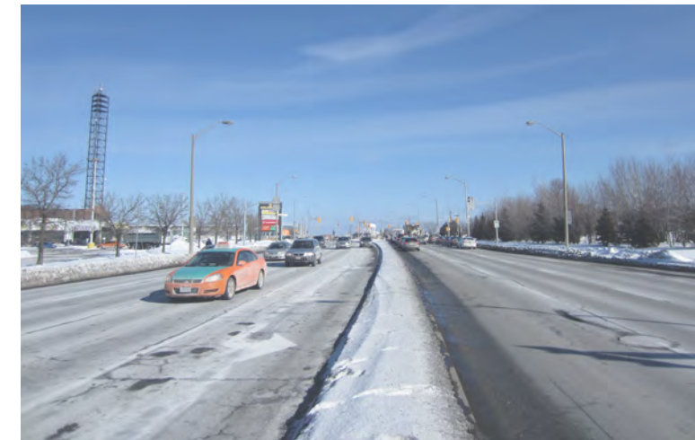
fig 3.3 Image of Eglinton Avenue's existing street condition near Victoria Avenue.
