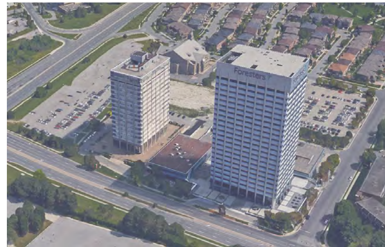
fig 3.65 Axonometric photo looking northeast at the office towers.
