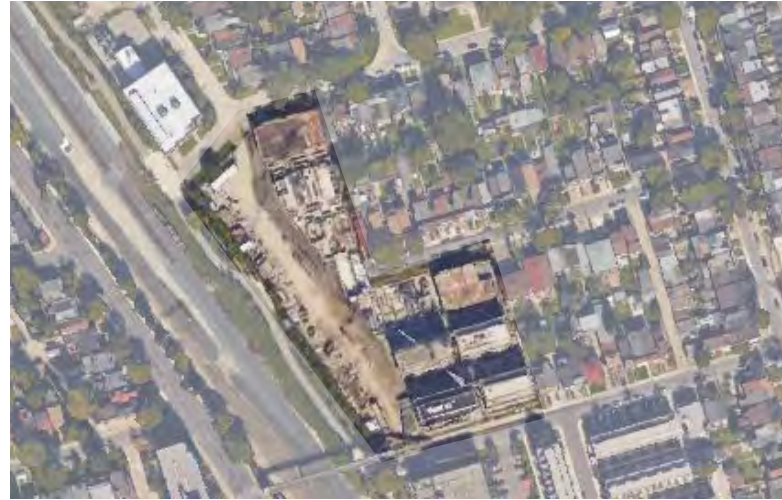
fig 3.100 Aerial photo of the project under construction.
