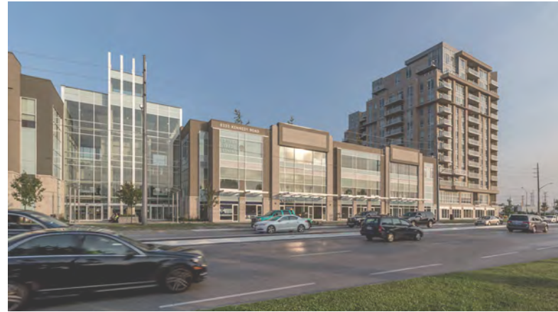
fig 3.57 Photo the main street's frontage and mid-rise tower looking south.
