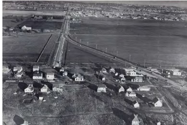
fig 2.6 Picture of the Golden Mile circa 1949 along Eglinton Avenue at Victoria Park Avenue with a munitions plant in the distance.
