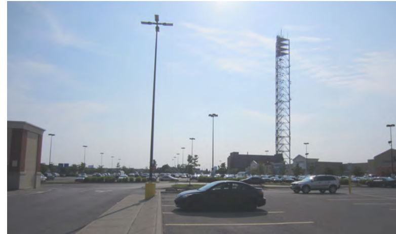
fig 2.3 Image of a typical Golden Mile site condition.
