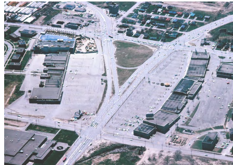
fig 4.41 Picture of Eglinton Avenue at Victoria Park and O’Conner Drive looking west in 1963.
