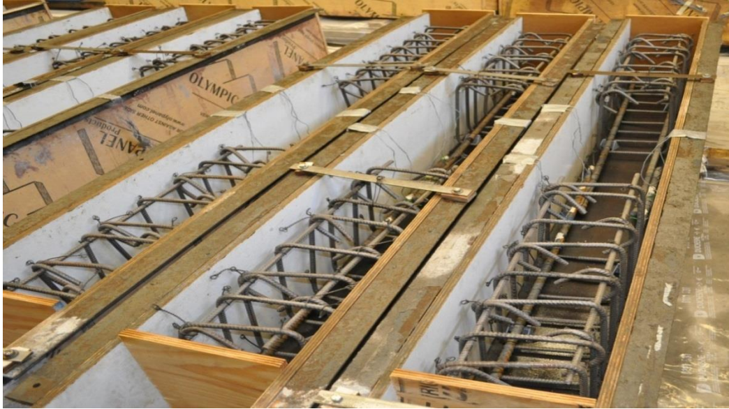
Figure 3.6 Cage inside formwork
