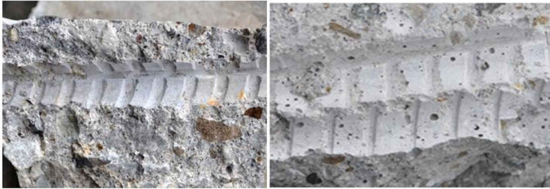
Figure 4.15 The interface of the concrete ahead of the steel bar ribs for the unwrapped beam
