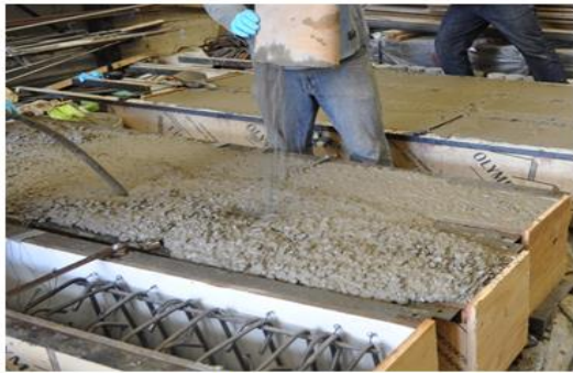
Concrete placing process
