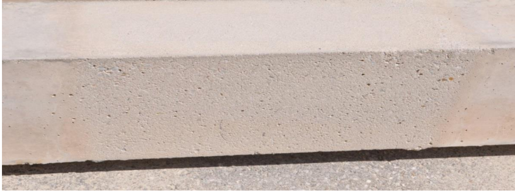
Figure 3.11 Concrete service after sandblasted
