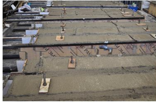
Concrete surface after finishing
