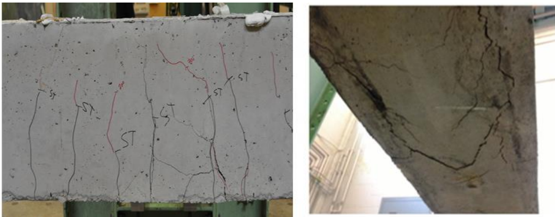
Figure 4.14 Flexural and splitting cracks on the unwrapped specimen
