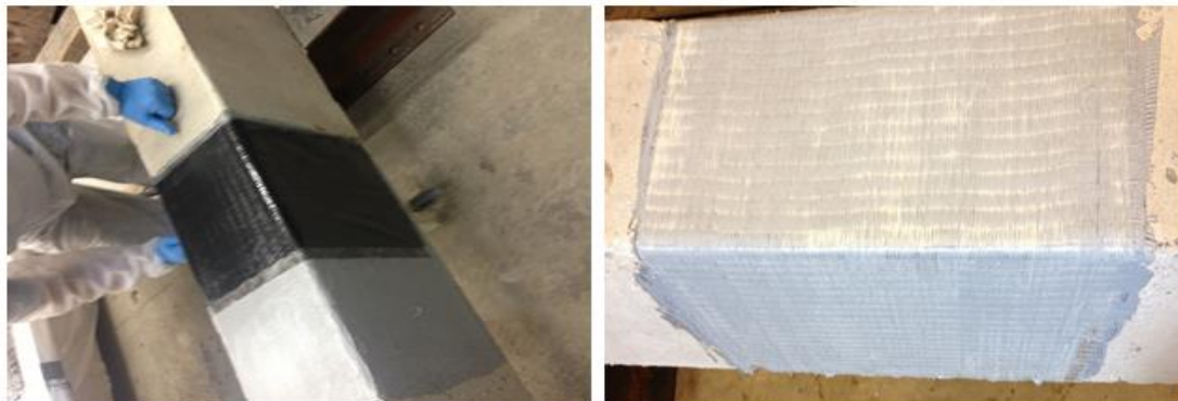
Figure 3.12 Installation of FRP wrapping sheets
