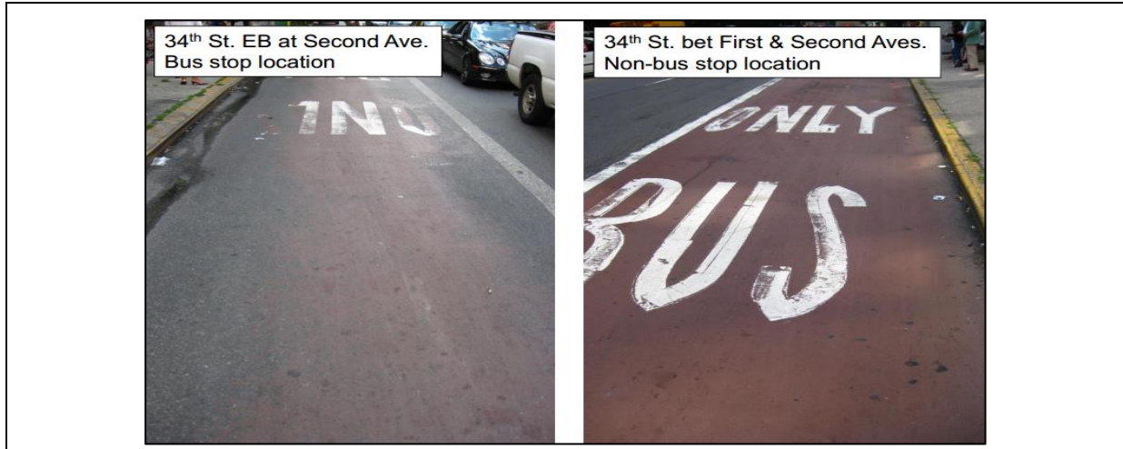
Figure 2-20 Effect of Stopping/Starting of Buses and Engine Heat Exposure (Carry, 2012)
