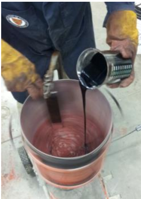
(c) Adding polymer modified asphalt binder
