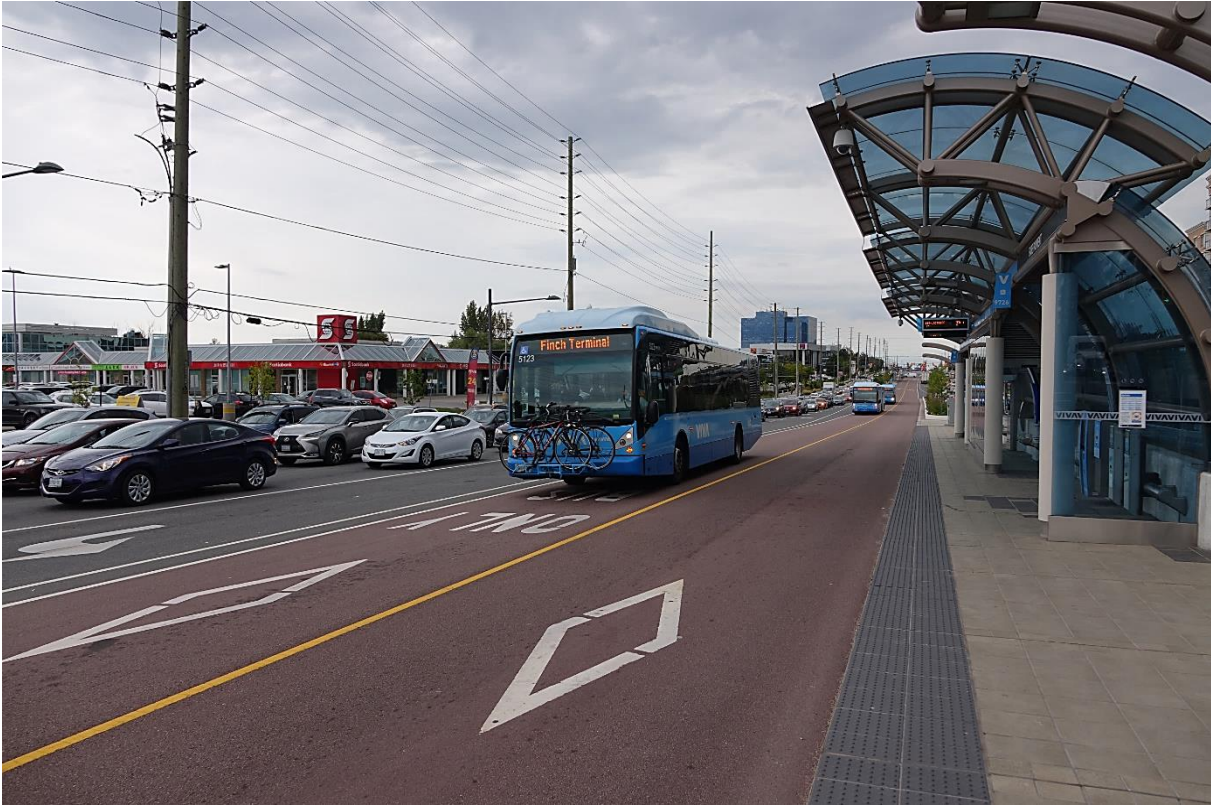
Figure 1-2 A section of Highway 7 BRT-Lane, York Region Ontario, August 2014
