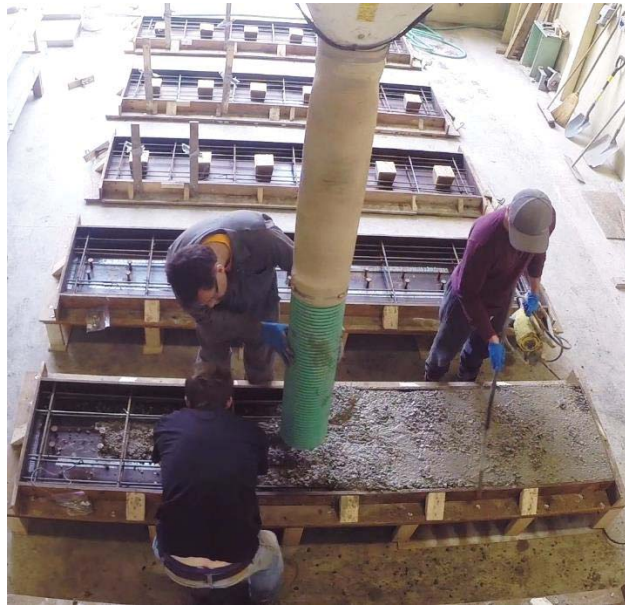
Figure 3-15: Concrete placement into a CIP specimen.
