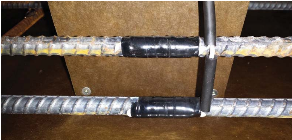
Figure 3-13: Top and bottom longitudinal reinforcement strain gauges prepared with a protective coating of rubber SB tape and electrical tape. Also included is the tubing providing the wire protection.
