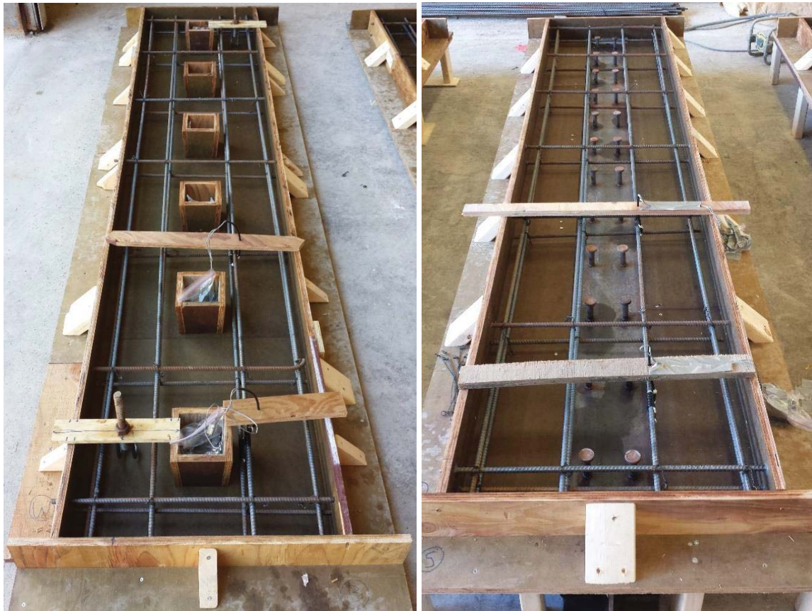
Figure 3-10: Formwork for the precast (left) and CIP (right) specimens.
