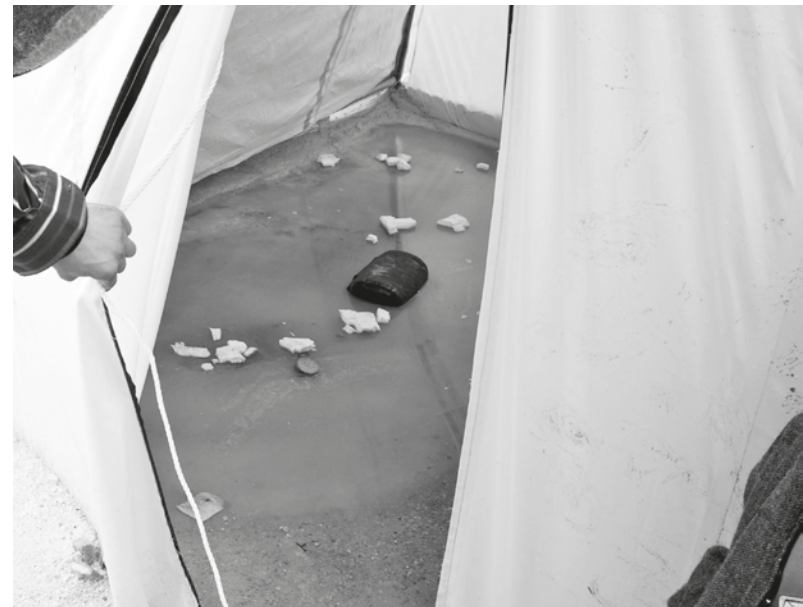
Fig 2.05 People abandon disaster-relief tents because of rain water leakage into their living area.
