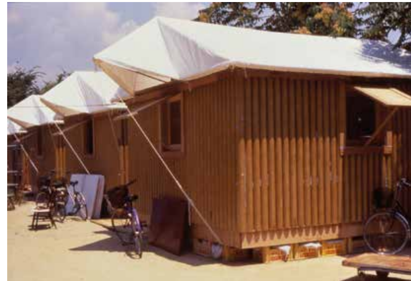
Fig 3.10 Paper log houses are temporary structures designed by Shigeru Ban after the 1995 earthquake in Japan. This shelter is built with recyclable paper tubes, donated beer crates loaded with sandbags, and tenting material for the roof. The units are dismantable and the materials can be recycled. 39 Although this project is designed for long term temporary use by disaster victims or refugees, it only meets the requirements of a short term temporary shelter by not being properly insulated, and lacking the most basic living conditions such as sanitary facilities and kitchen. Furthermore, since paper log houses are not mobile, they still involve dealing with land rights and official permissions which complicates the construction process.
