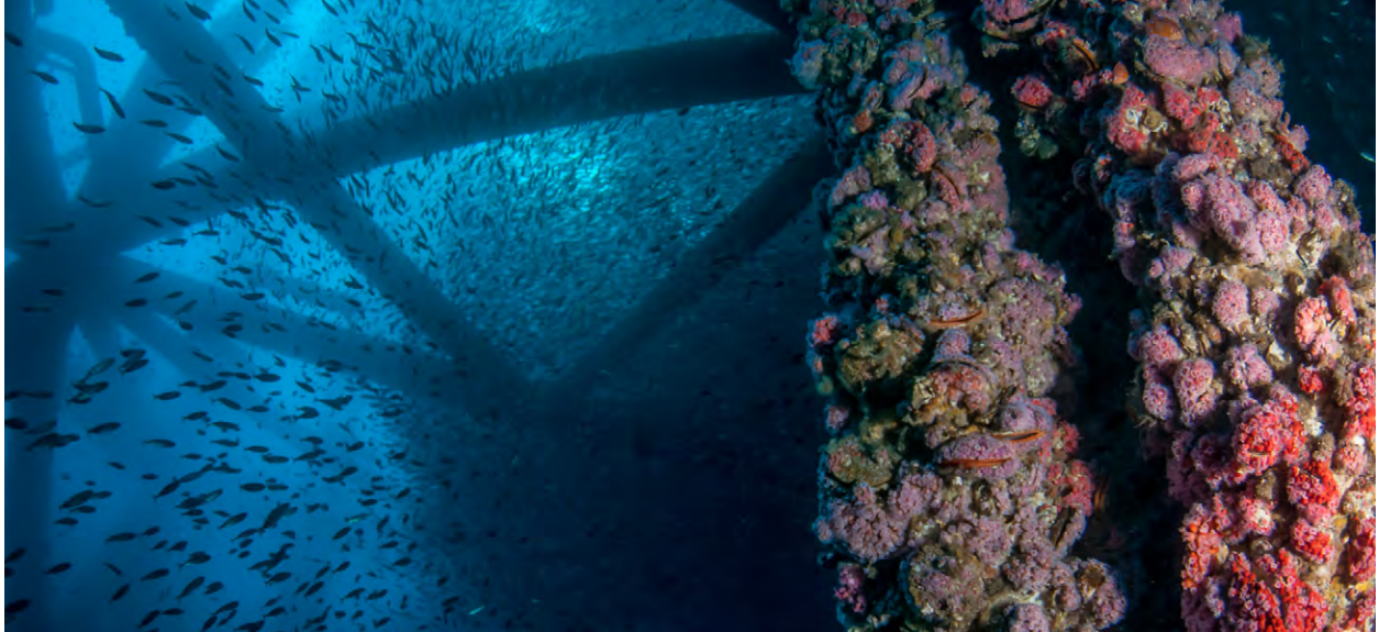
Figure 26: Structure's columns covered in a thick layer of life
