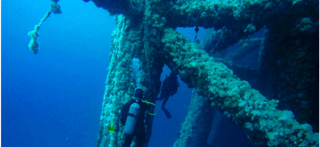
Figure 28: Divers investigating the structure
