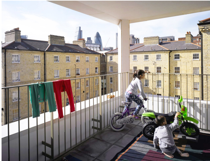
Fig. 3.15. View of corner balcony of one of the units.
