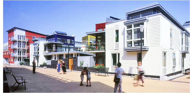
Fig. 3.18. Exterior of building from street.
