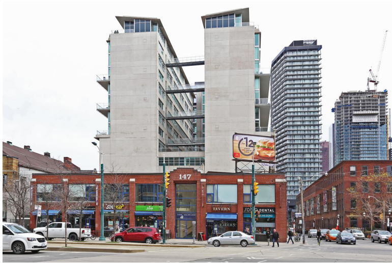
Fig. 3.59. West building facade, showing exterior bridges on every second floor.
