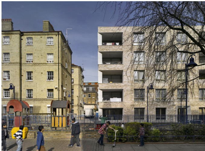
Fig. 3.16. View of building from central playground.
