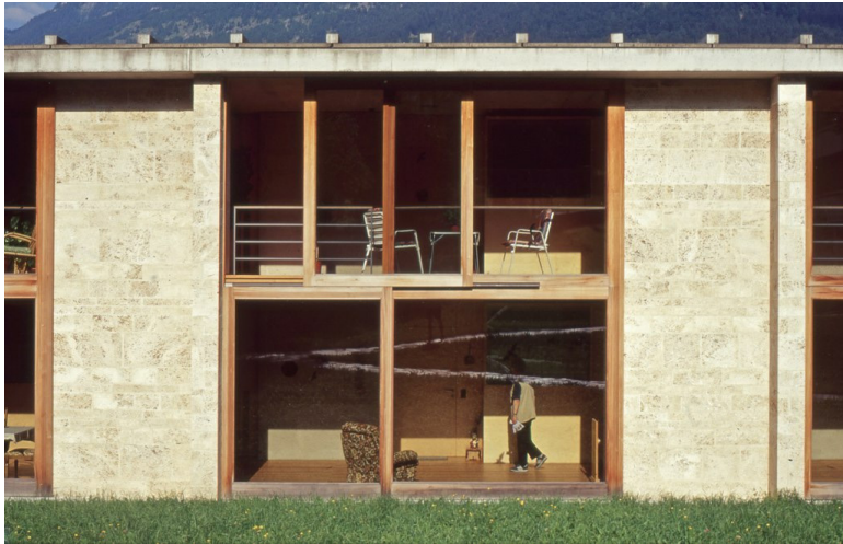
Fig. 3.32. View of the single-loaded corridor from the exterior of the building, with large, east-facing windows.
