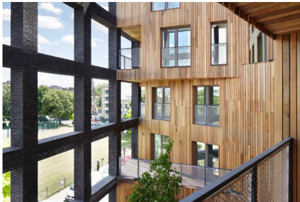
Fig. 2.15. Wenlock Cross, the first ten-storey building to be built using CLT. Designed by Hawkins/Brown, the building consists of 50 units ranging in size from one to three bedrooms.
