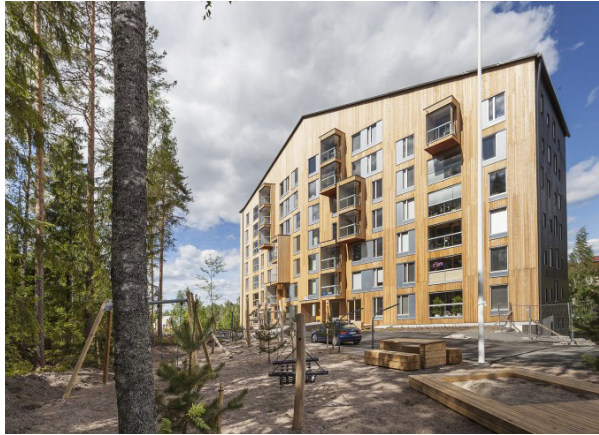
Fig. 2.14. Puukuoka, an eight-storey housing block, design by the Finnish firm OOPEAA and built using CLT. The project was planned in collaboration with the City of Jyväskylä to ensure the affordability of its units.
