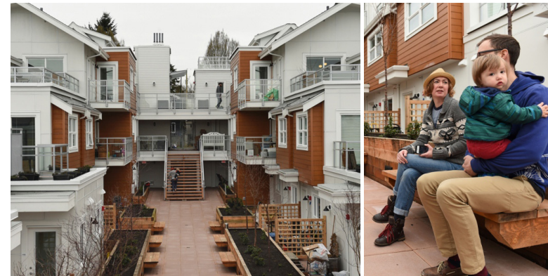
Fig. 1.20. Vancouver’s first co-housing complex.
