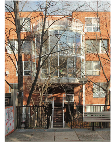
Fig. 3.55. View of third floor common area and its connection to the courtyard.
