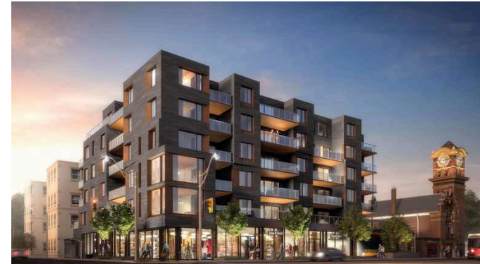
Fig. 5.03. Rendering of Heartwood the Beach condominium, a project by Quadrangle for the developers Fieldgate Urban and Hullmark Development, expected to be completed in spring of 2017. This is one of the first six-storey wood building to be built in Toronto since the Building Code amendment.
