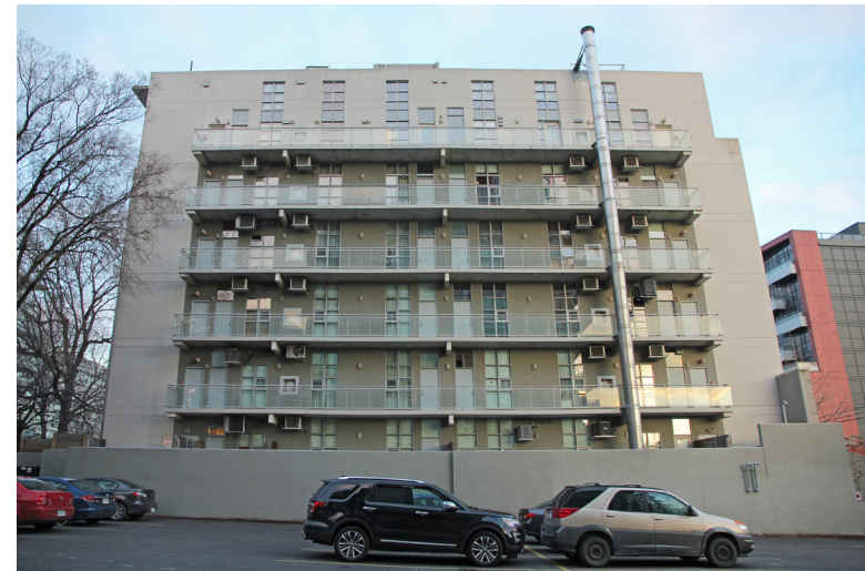
Fig. 3.57. West building facade, showing exterior corridor on each floor.
