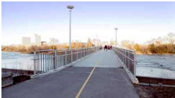
1.24 Adawe crossing looking East - December 2015
