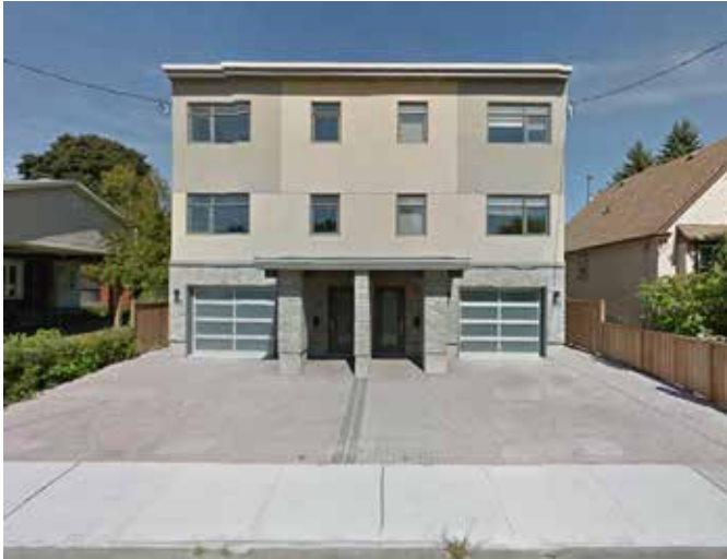
3.21 Semi-Detached infill. 135 Prince Albert St, Overbrook.
