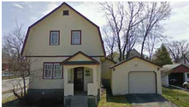
1.21 Pre-war dwelling with detached garage 158 King George, Overbrook
