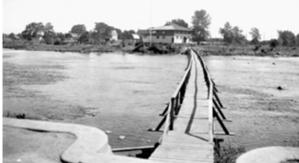
1.25 Seasonal footbridge looking East - Undated
