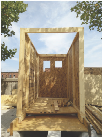
More walls were added,
