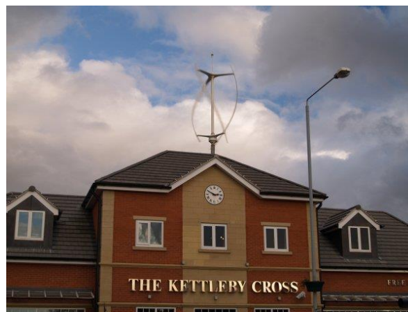
Figure 1.5: Vertical wind turbine on the roof of Witherspoon's pub known as "The Kettleby Cross" in Melton Mowbray [10].
