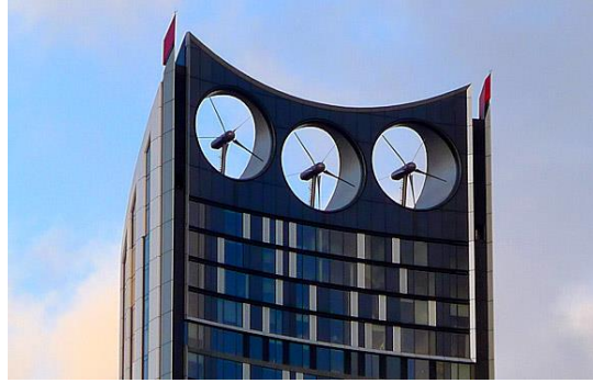
Figure 1.4: Wind turbines in the Strata Tower in London, UK [9].
