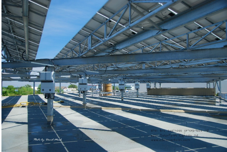
Figure 5.6 Suspended Panel System (SolarForm, 2016)
