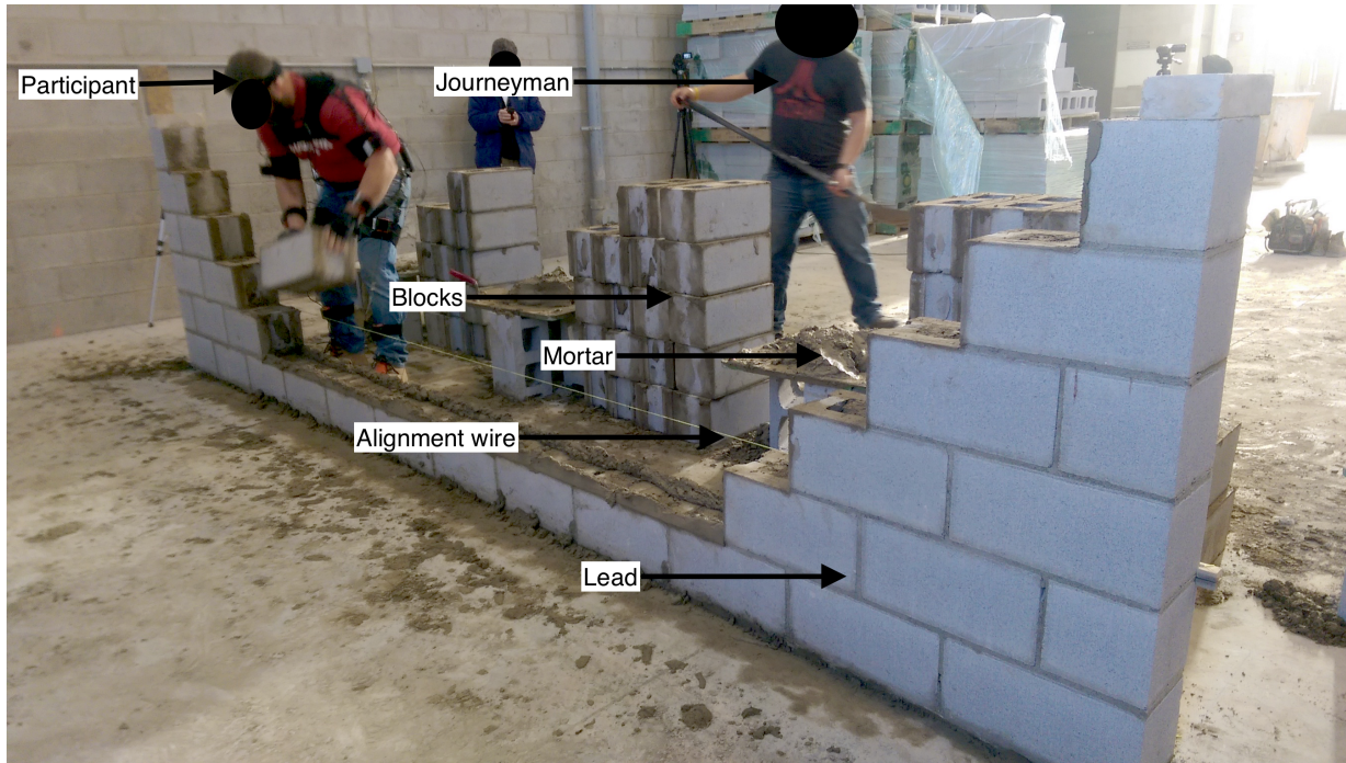
Figure 5.1: Lead wall built to guide participants.
