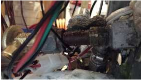
Fig. 13 TXV without frost
