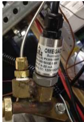
Fig. 6 Thermocouple & pressure transducer
