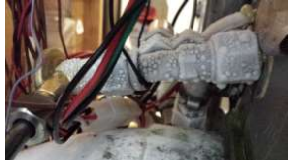
Fig. 14 TXV with frost
