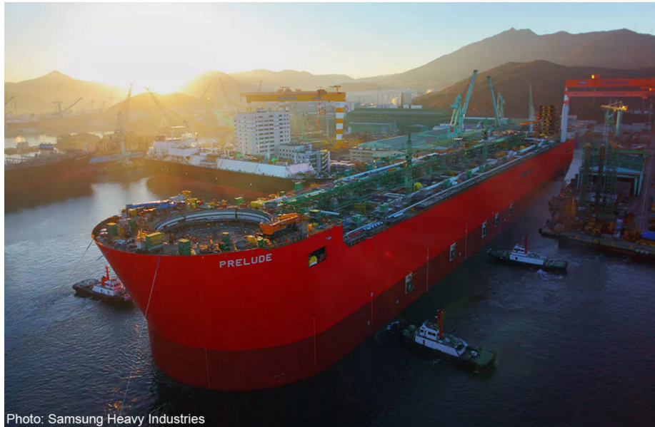
Figure 1.1: The world's first floating liquefied natural gas facility [1].
