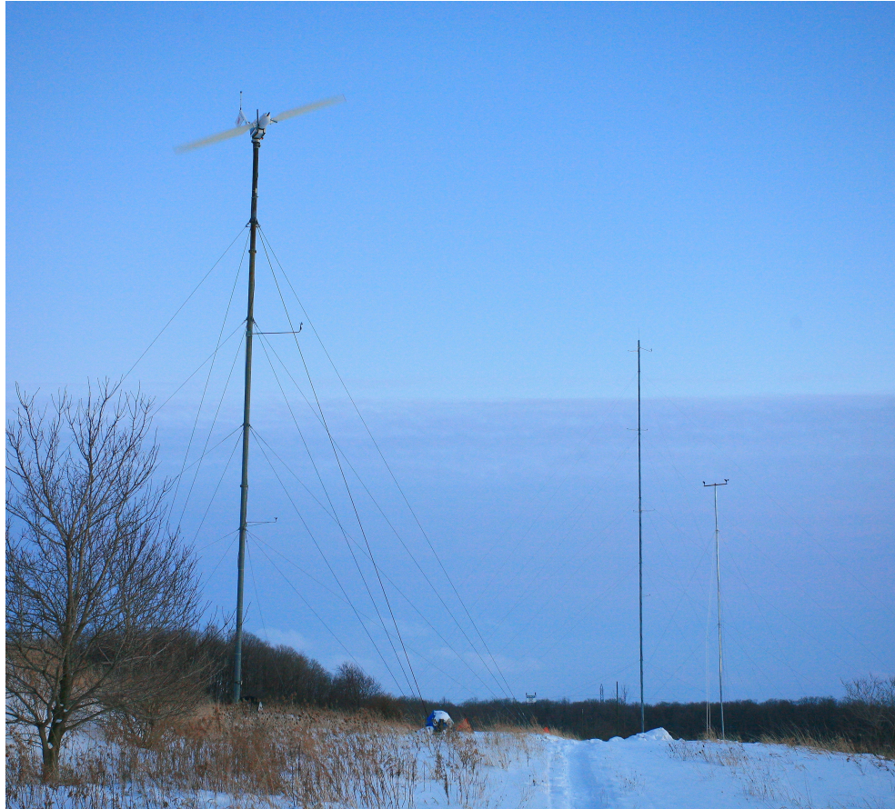
Figure 3.18: View of the Wind Energy Group wind turbine test site from the north. For the towers shown, from left to right: wind turbine tower, 50 m MET tower, 10 m MET tower
