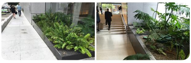
**FIG.3.7:** The San Francisco Public Utilities Commission has installed living machines in their headquarter in San Francisco and the system is able to treat and return up to 5,000 gallons of wastewater per day for non-potable water use in the building. The photos above show the outdoor (left) and indoor(right) wetland cells of the living machine.<sup>8</sup>
