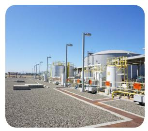
FIG.3.10: Tanks outside the facility for storage of purified water
