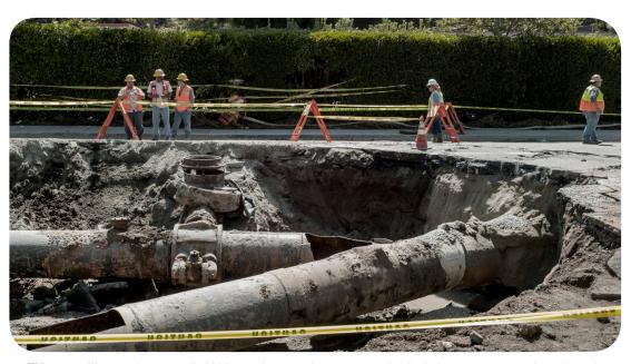
FIG.2.20: Water mains normally hidden underground were exposed only during system upgrade and repair.
