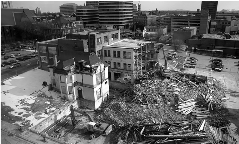
Fig. 2.15 Demolition of the John Forsyth Shirt Factory
