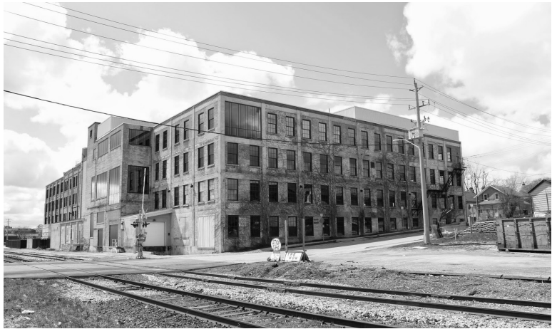
Fig. 2.14 Former Boehmer Box Factory
