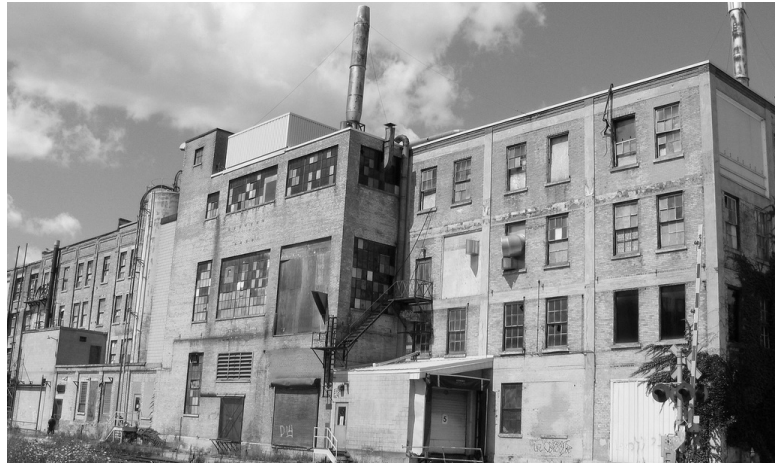
Fig. 2.17 Former Dominion Tire Plant
