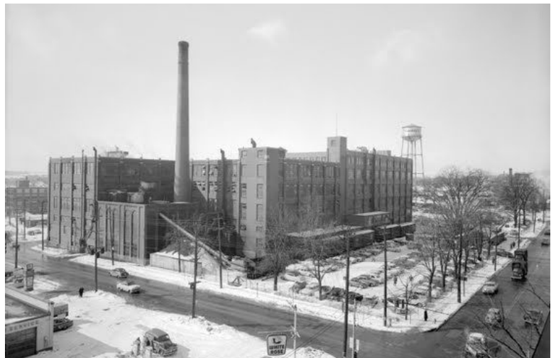
Fig. 2.1 1959 B.F. Goodrich Plant at King & Victoria, Kitchener
