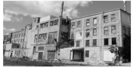
2 Dominion Tire Plant
