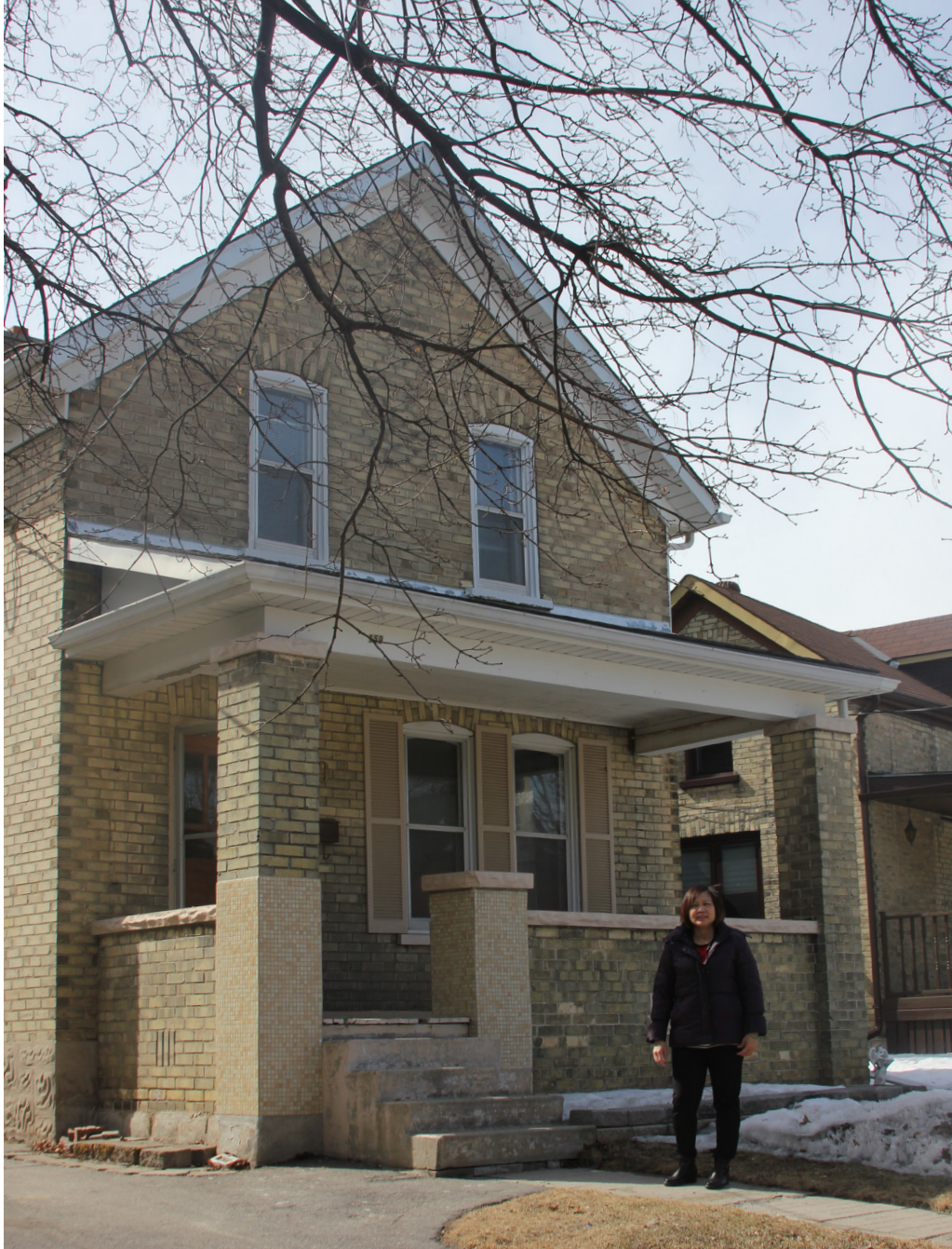
Fig. 3.1 Renovation of Personal Kitchener Residence
