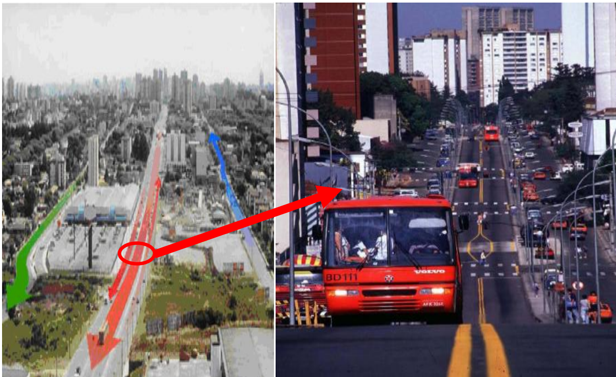
Figure 8 The central avenue in the trinary road system also consists of three roads. (Jian, 2010)
