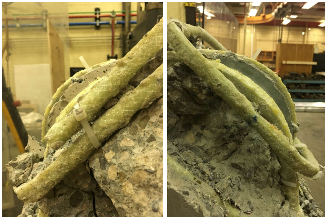
Figure 4.21: Slip of Longitudinal Bars towards Adjoining Members, CA-3-6
