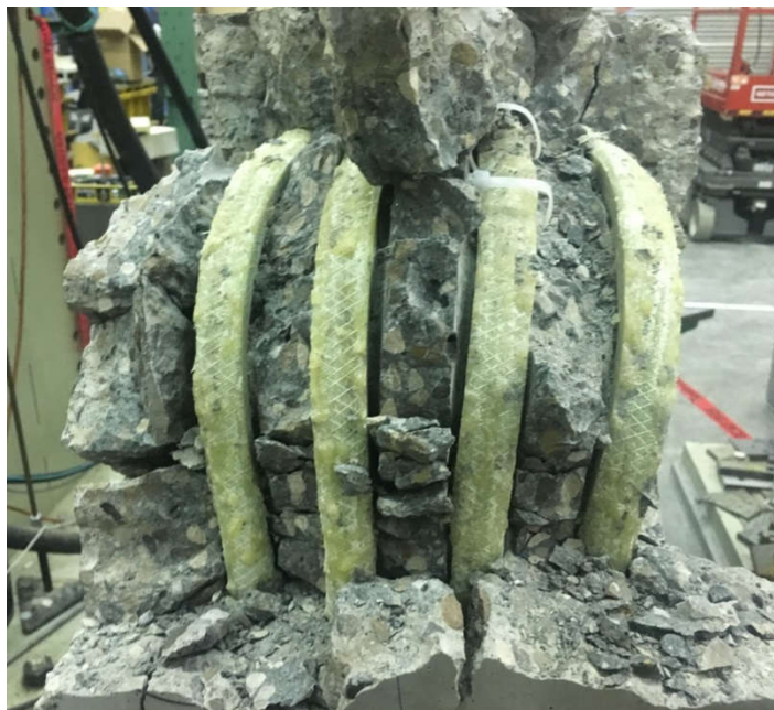
Figure A.13: Back Side of Failed Joint, UA-4-6
