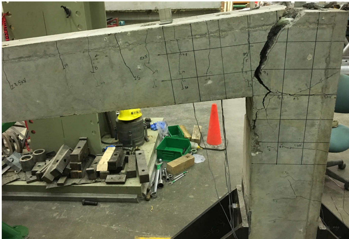
Figure 4.7: Crack Patterns on East Face, UA-2-6
