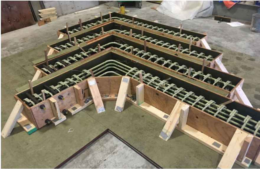
(b) Reinforcement Cage in Assembled Formwork
