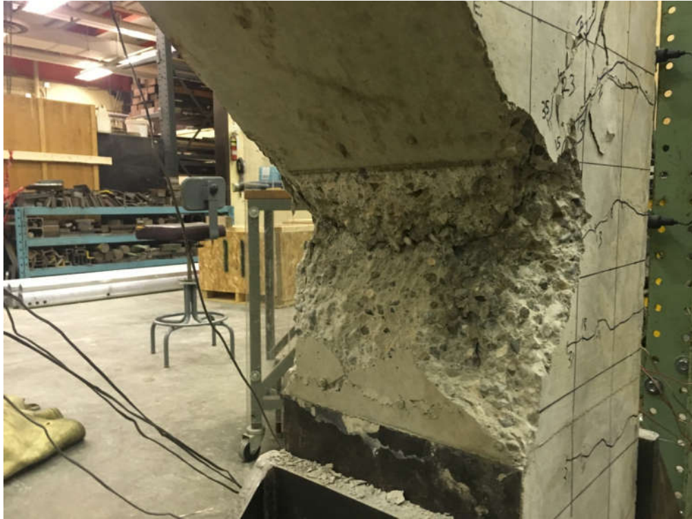
Figure A.56: Extent of Crushing on Interior Corner, CB-3-6
