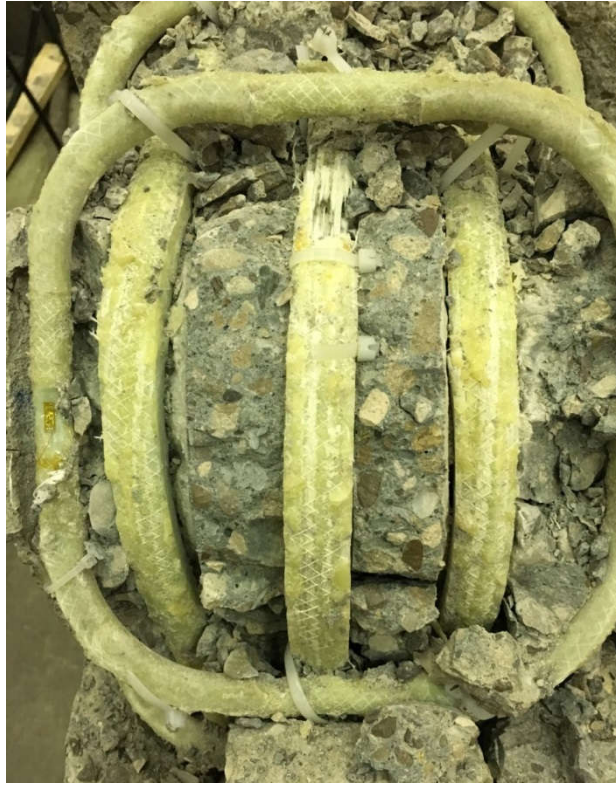
Figure A.44: Bar Rupture and Bar Shifting, CA-3-6
