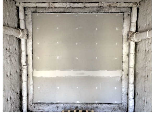
Figure 7.8: Finished wall, exposed side, dried and sanded.
