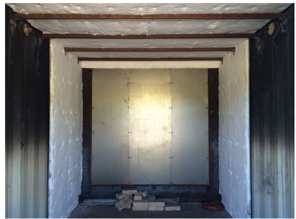
Figure 4.6: Insulation panels installed on the compartment walls.
