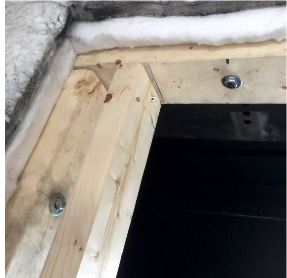
Figure 7.2: Frame insulation and mounting details.
