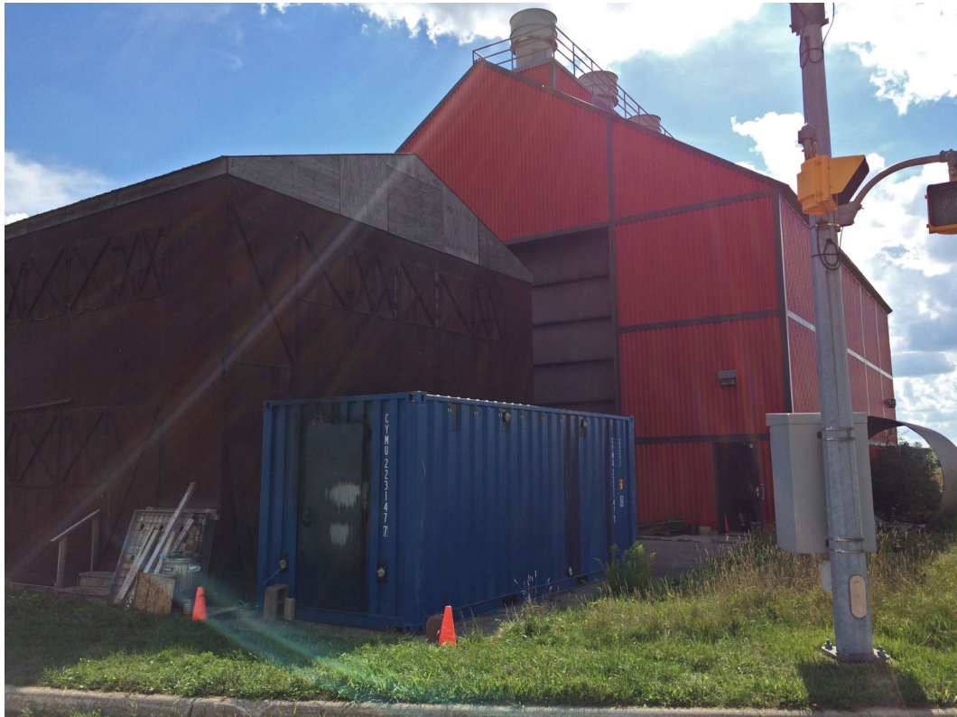
Figure 4.3: Fire test apparatus installed on site.
