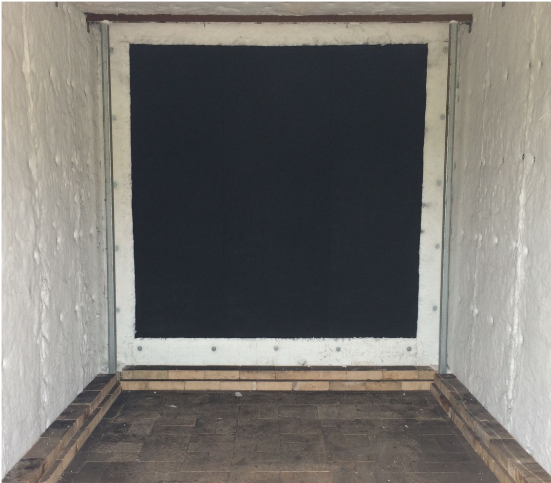
Figure 5.7: Steel wall surface preparation (coating).
