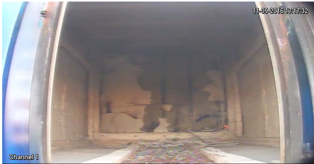
Figure 7.47: Real wall test #5, fire-side camera, end-of-test.
