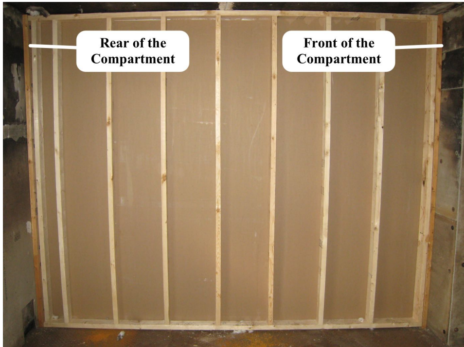
Figure 3.4: Stud wall being constructed, unexposed side of the wall.
