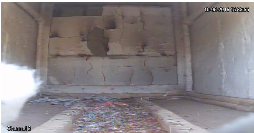
Figure 7.12: Real wall test #1, fire-side camera, 79.5 min.
