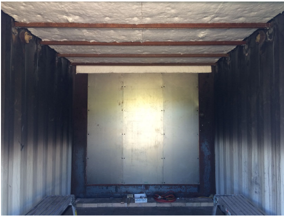
Figure 4.5: Insulation panels installed on the compartment ceiling.
