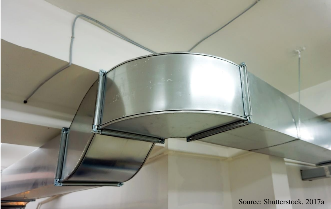
Figure 34: Ventilation Ducts made up of Galvanized Sheets
