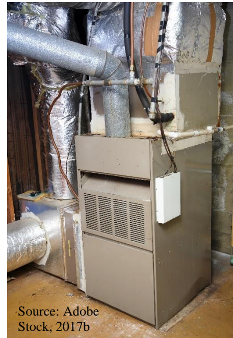
Figure 47: Natural Gas Furnace with Duct Work
