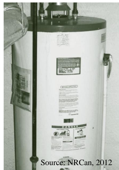
Figure 54: Conventional Gas Fired Water Heater
