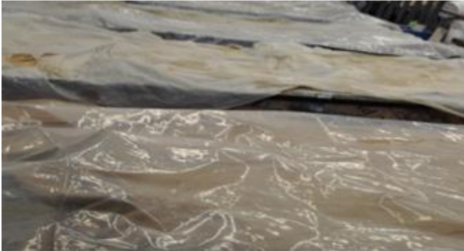
Concrete curing (burlap and plastic)
