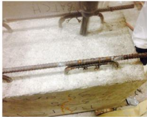
Figure 3.10 Surface roughening of region to be repaired
