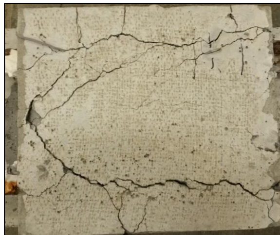
Figure 6.2 Bottom face bond splitting cracks for an unconfined beam
