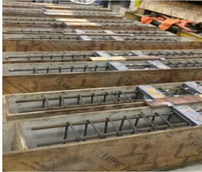
Figure 5.8 Reinforcement cages placed inside the formwork
