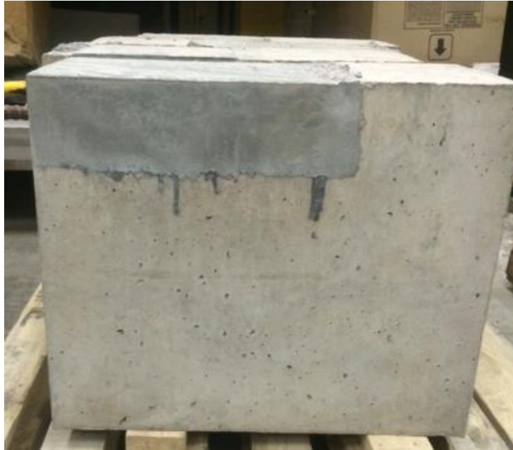
Figure 3.11 Completed specimen after applying partial depth repair concrete
