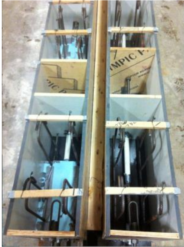
Figure 3.8 PVC pipes and foam installation in formwork
