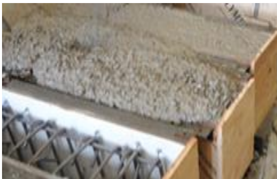
Concrete placement
