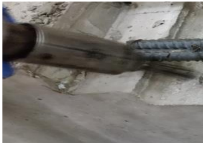
Figure 5.10 Roughening the substrate concrete with needle peener
